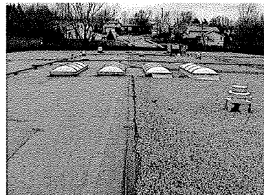
A2: Cottonwood Roof
