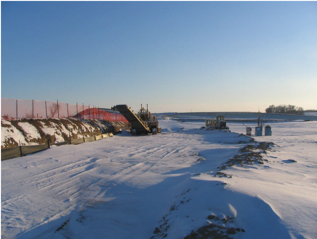
Elementary #24 @ 198 th Street looking South – December 6, 2005
