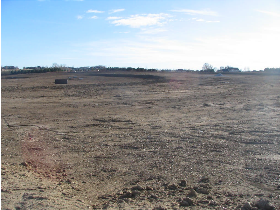
Elementary #25 Building location looking South – January 04, 2006
