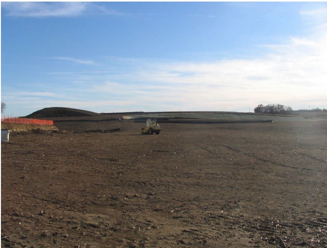
Elementary #24 @ 198 th Street looking South – January 04, 2006
