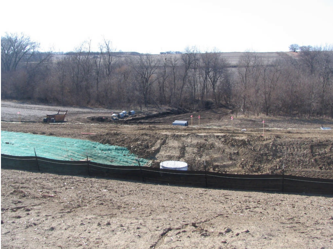
Elementary #24 @ Storm Sewer Drainage work @ creek – March 11, 2006
