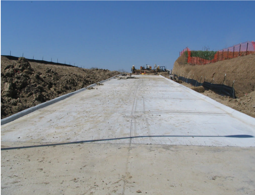
Elementary #24 Public street progress at J Street – April 10, 2006
