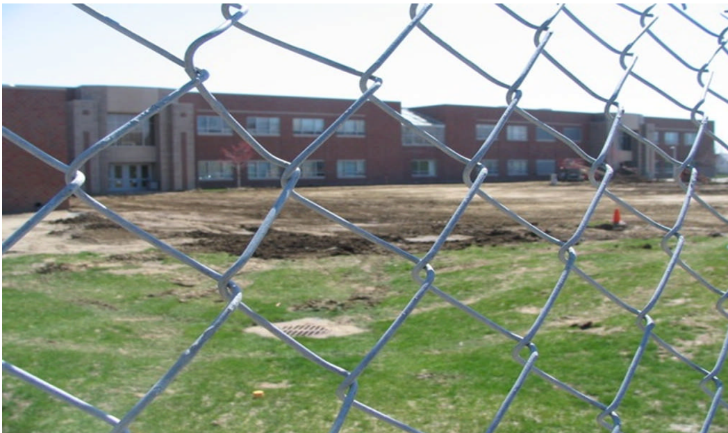
West High School Earthwork in progress – April 10, 2006
