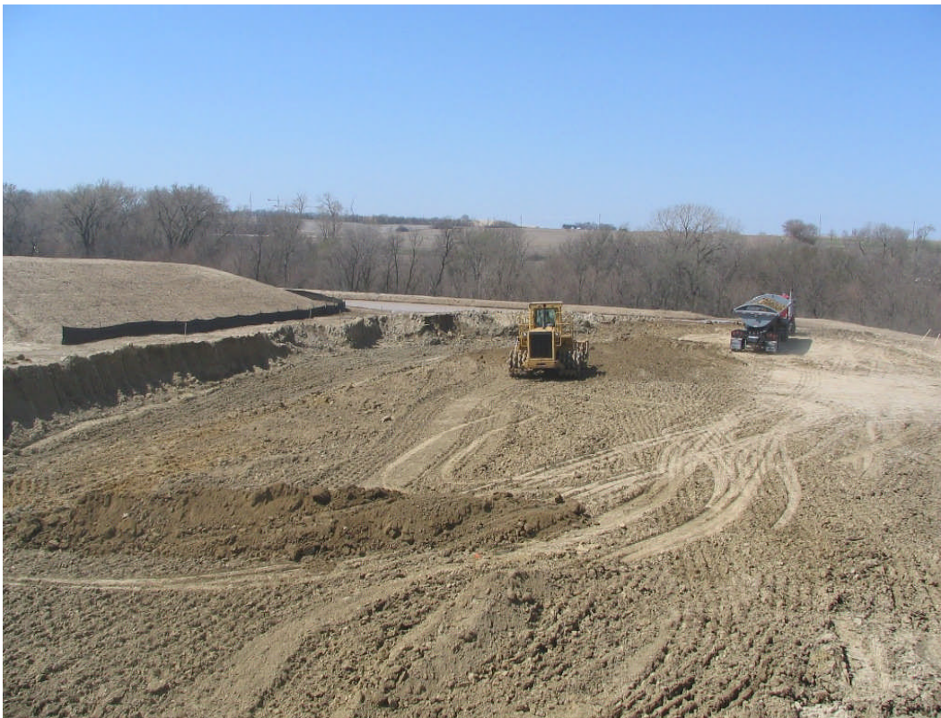
Elementary #24 Building Footing excavation work – April 10, 2006
