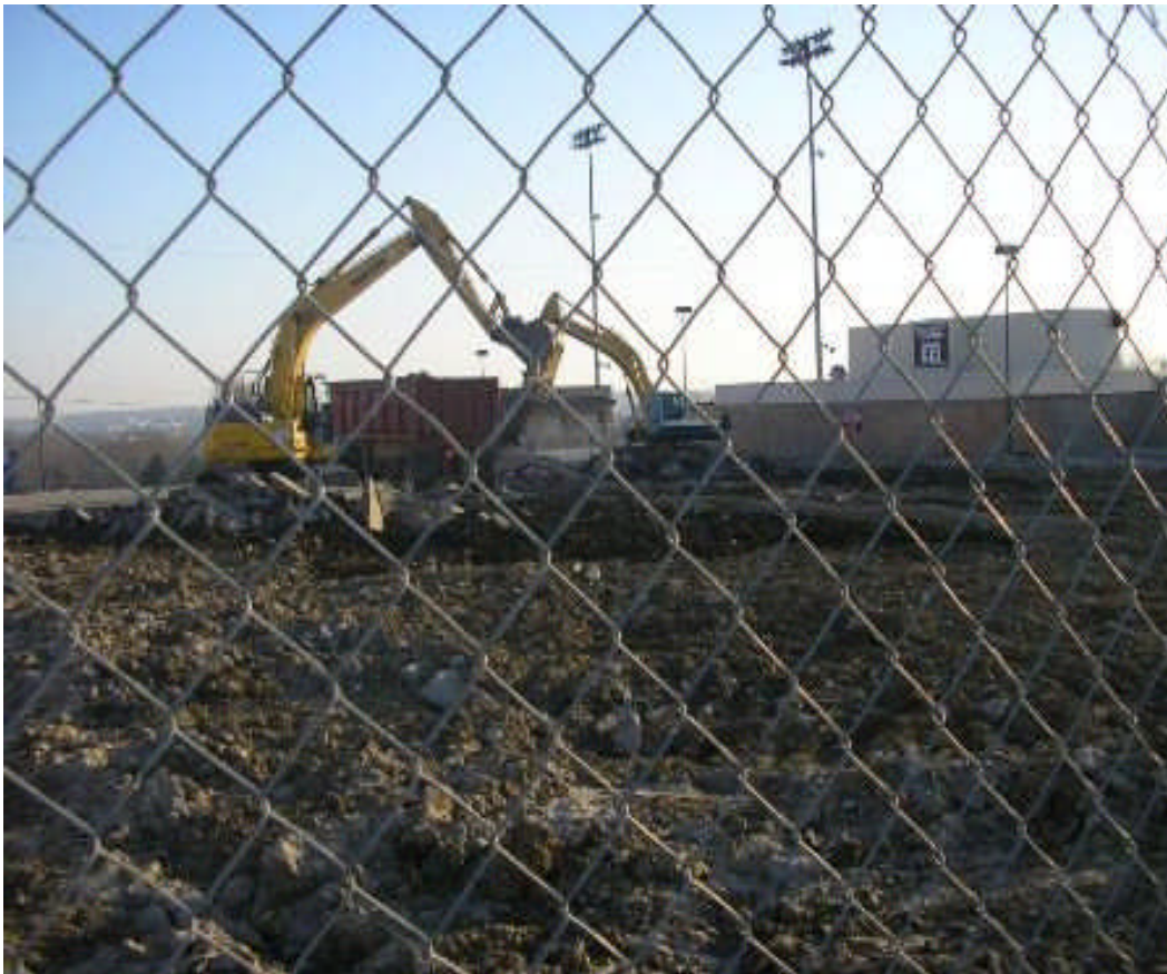
South High School Parking lot removal – April 10, 2006
