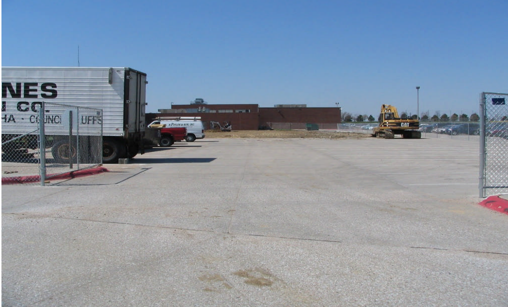
North High School Building addition parking lot removal – April 10, 2006
