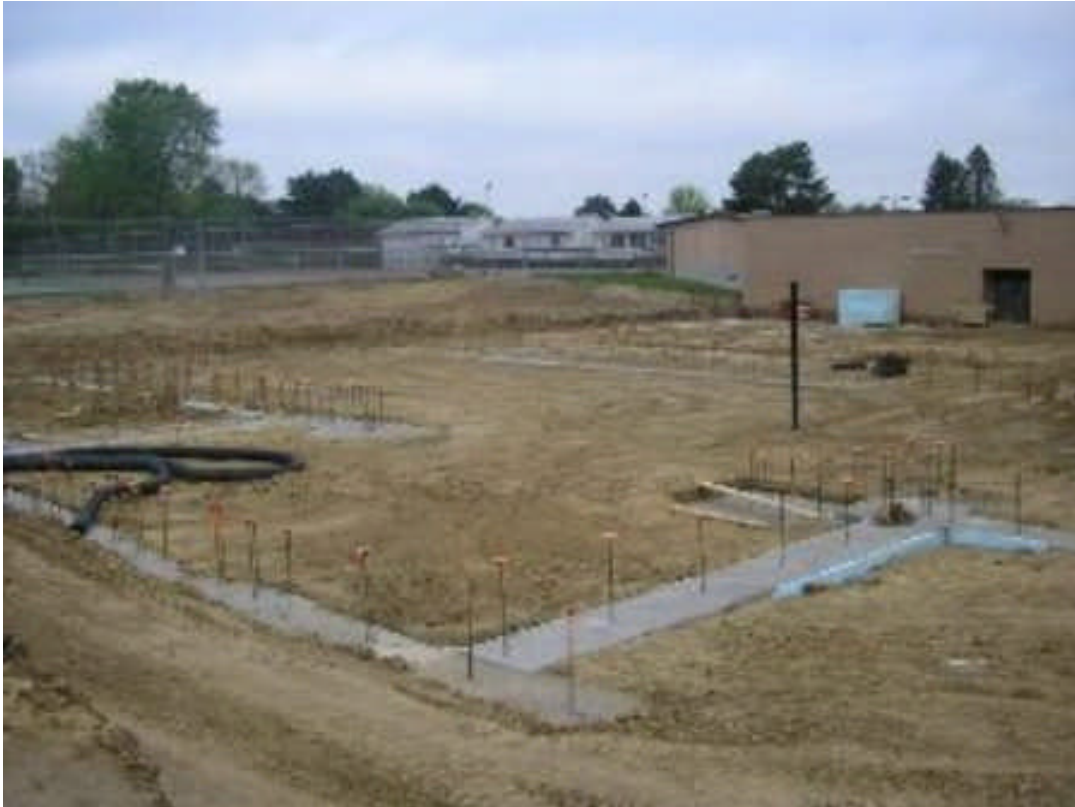
South High School - foundation work complete at addition - May 8, 2006
