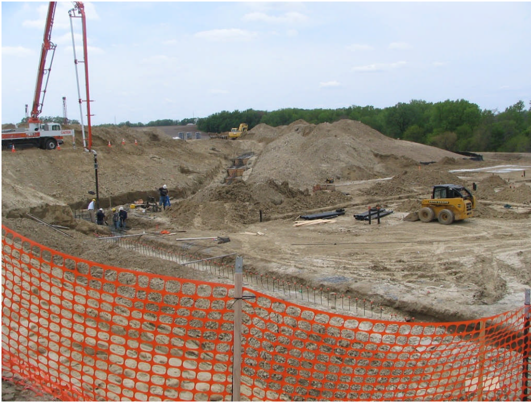
Elementary #24 – building footing excavation work – April 10, 2006
