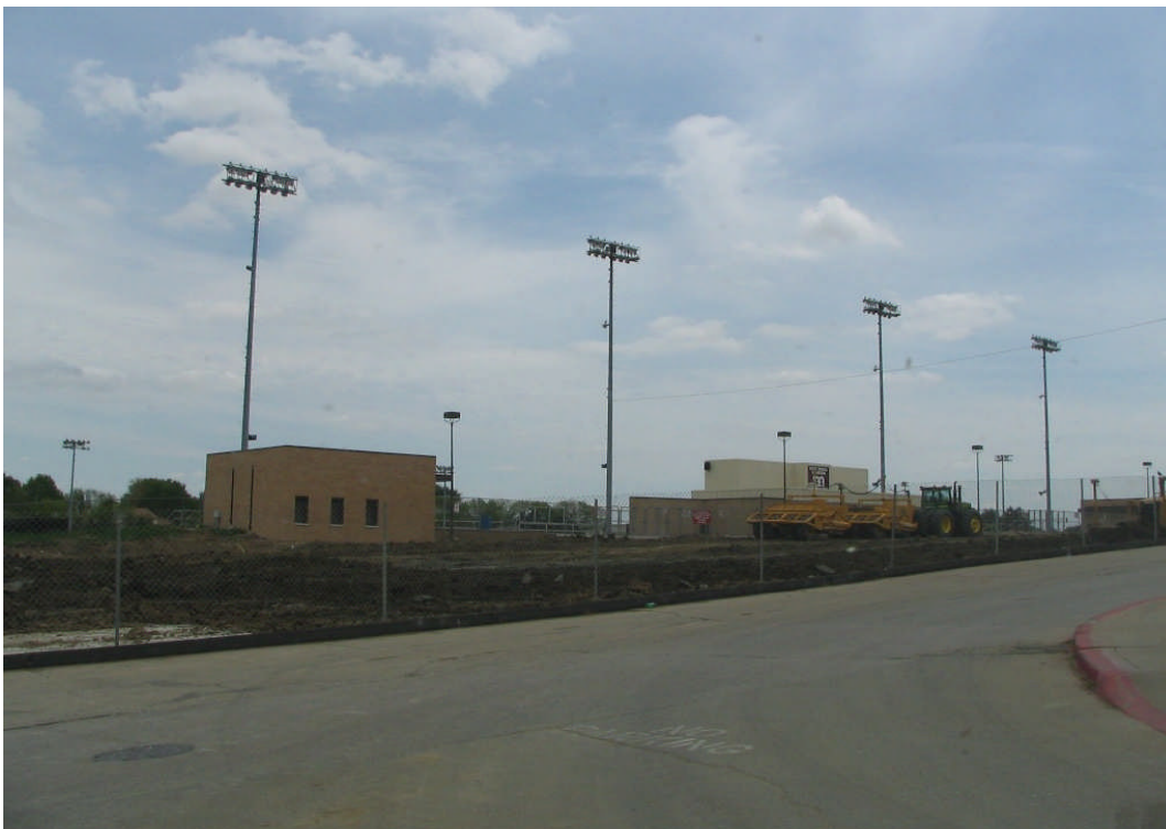
South High School - parking lot final grading (East side) – May 8, 2006
