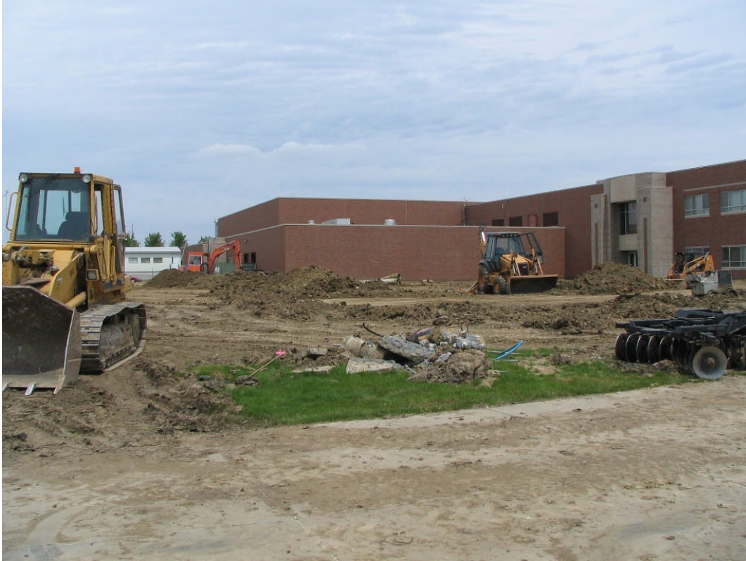
West High School - site utilities work in progress - May 8, 2006
