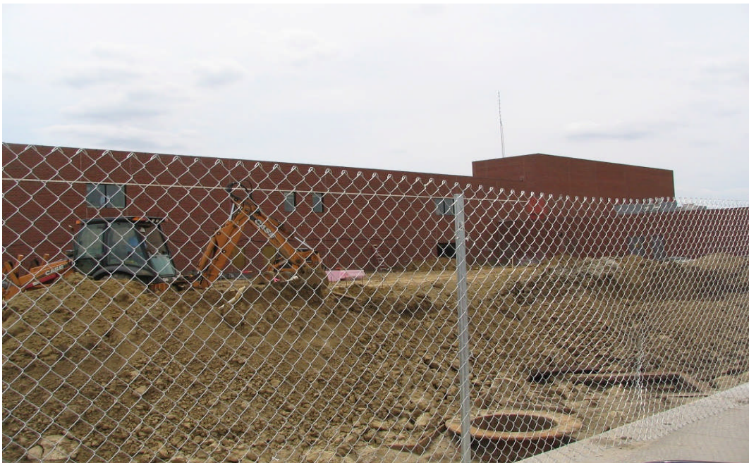
North High School - underground utility work at addition in progress - May 8, 2006
