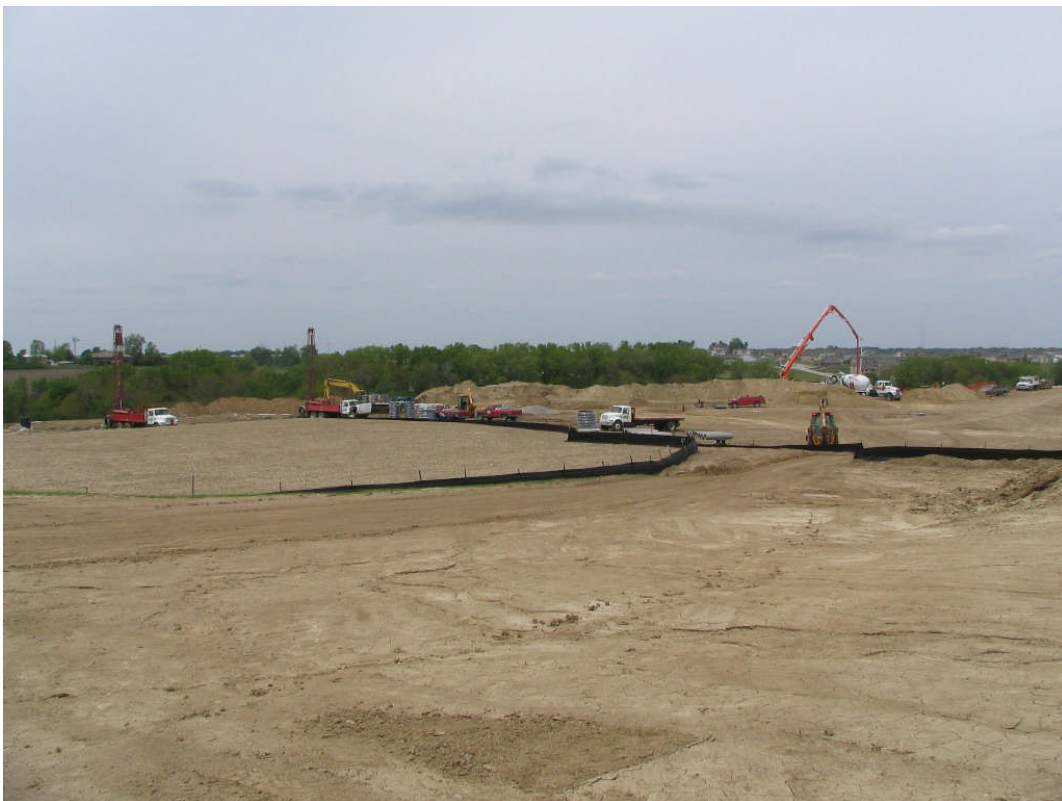
Elementary #24 - well field installation in progress – May 8, 2006
