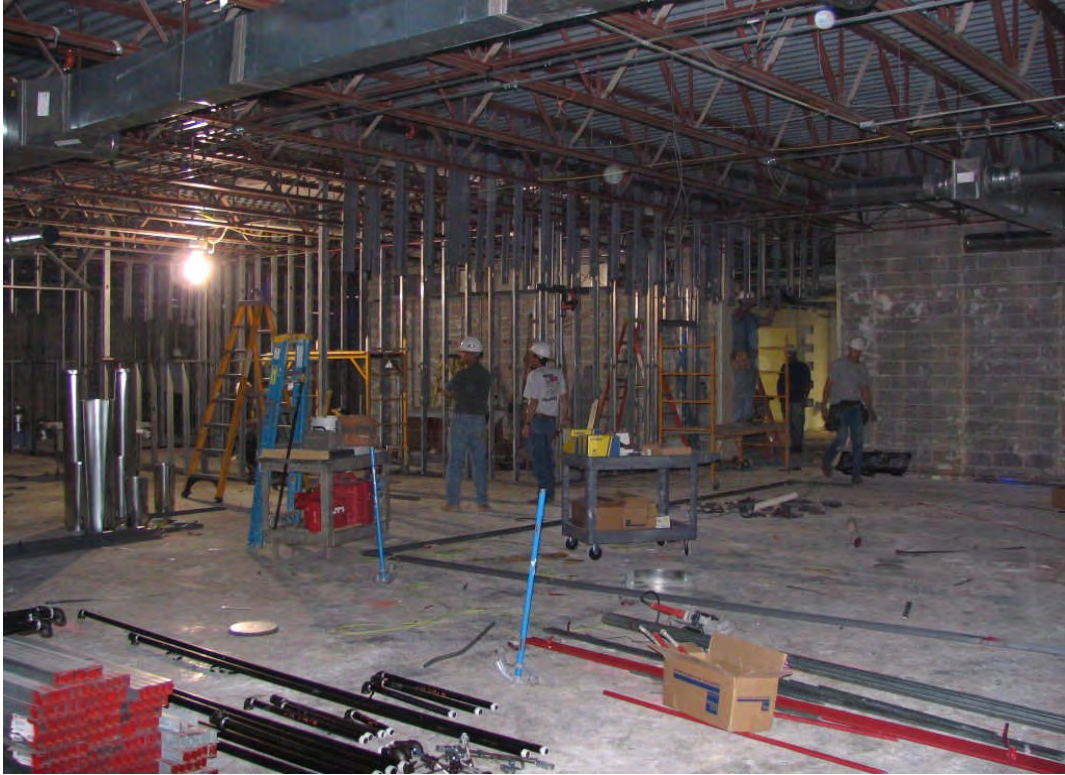
Ackerman Elementary – Demolition & wall construction in progress – June 12, 2006
