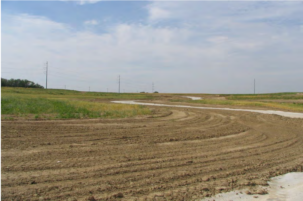
Elementary #25 – Street installation in progress – June 12, 2006
