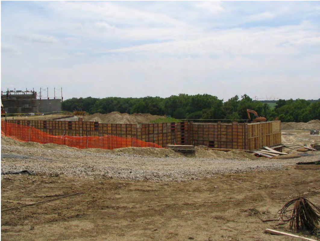
Elementary #24 – Masonry & Foundation wall work in progress – June 12, 2006
