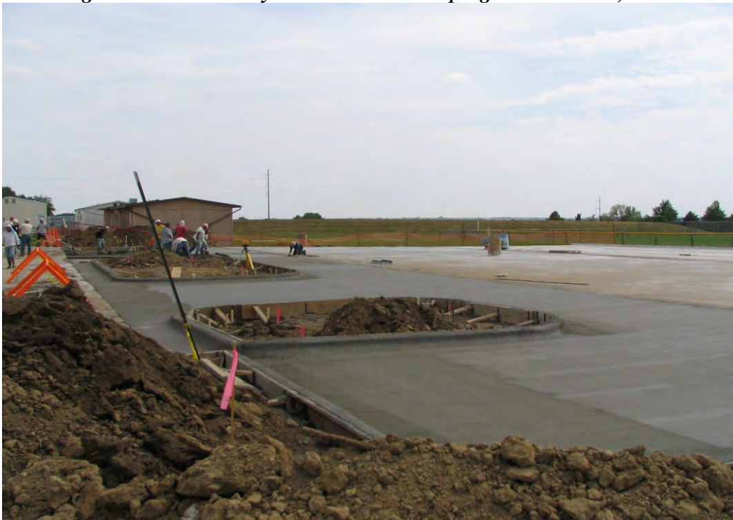
North High School – Northwest parking lot continues– June 12, 2006
