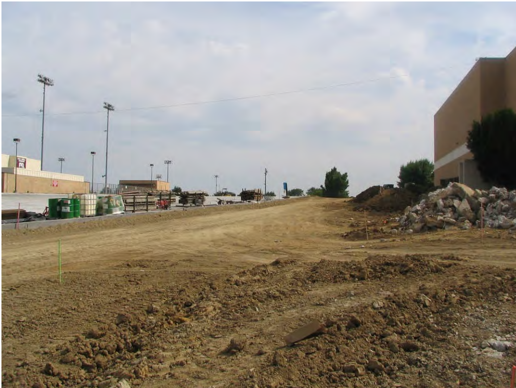
South High School – East parking lot final grading (West side) – June 12, 2006
