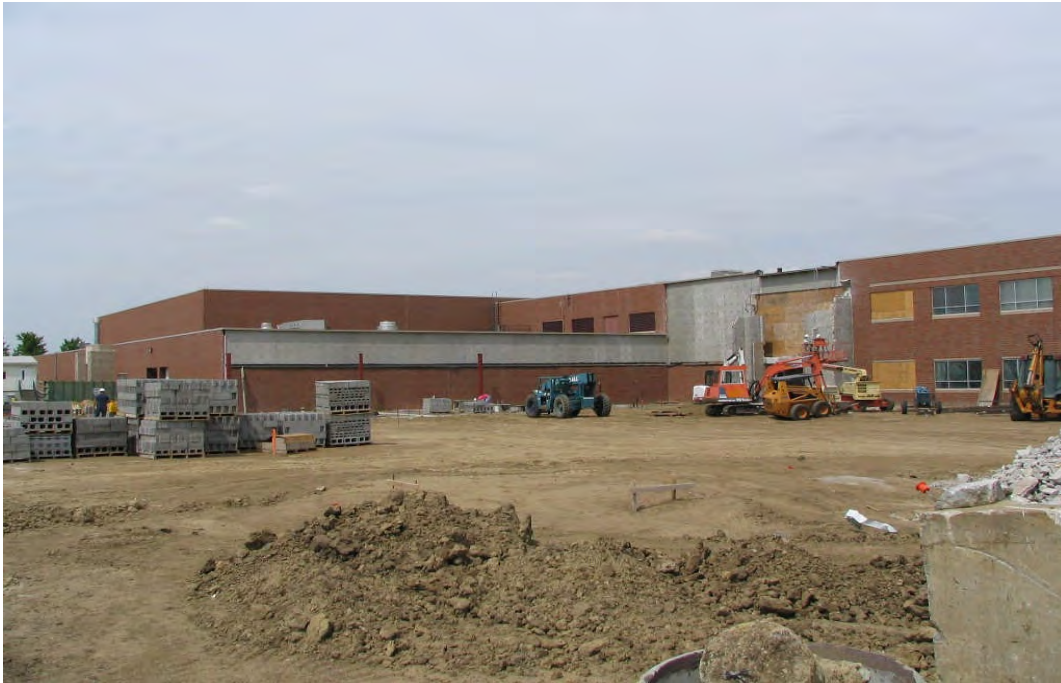
West High School – Masonry work at west addition in progress – June 12, 2006
