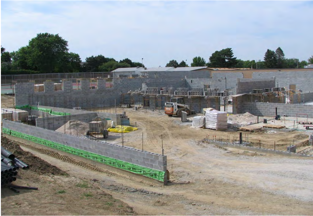
South High School - Masonry work continues at addition – June 12, 2006
