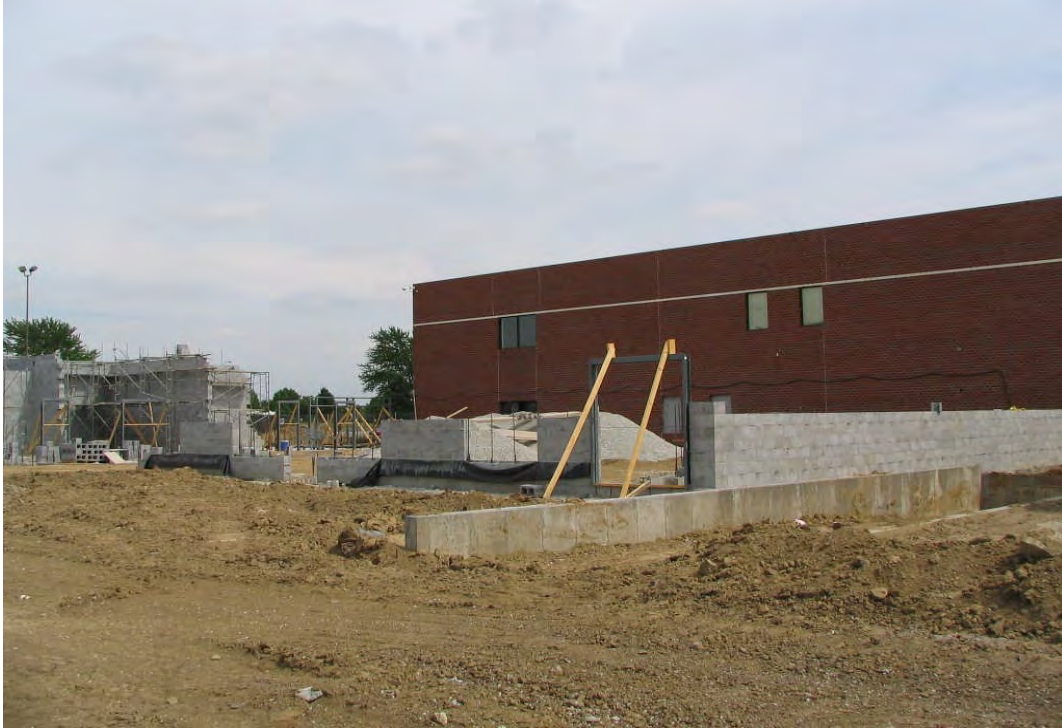
North High School – Masonry work at addition in progress – June 12, 2006
