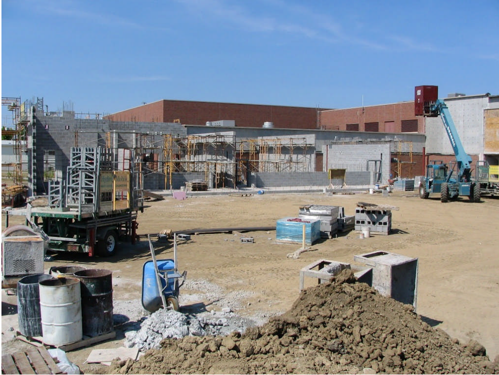
West High School – Building Addition (July 5, 2006)
