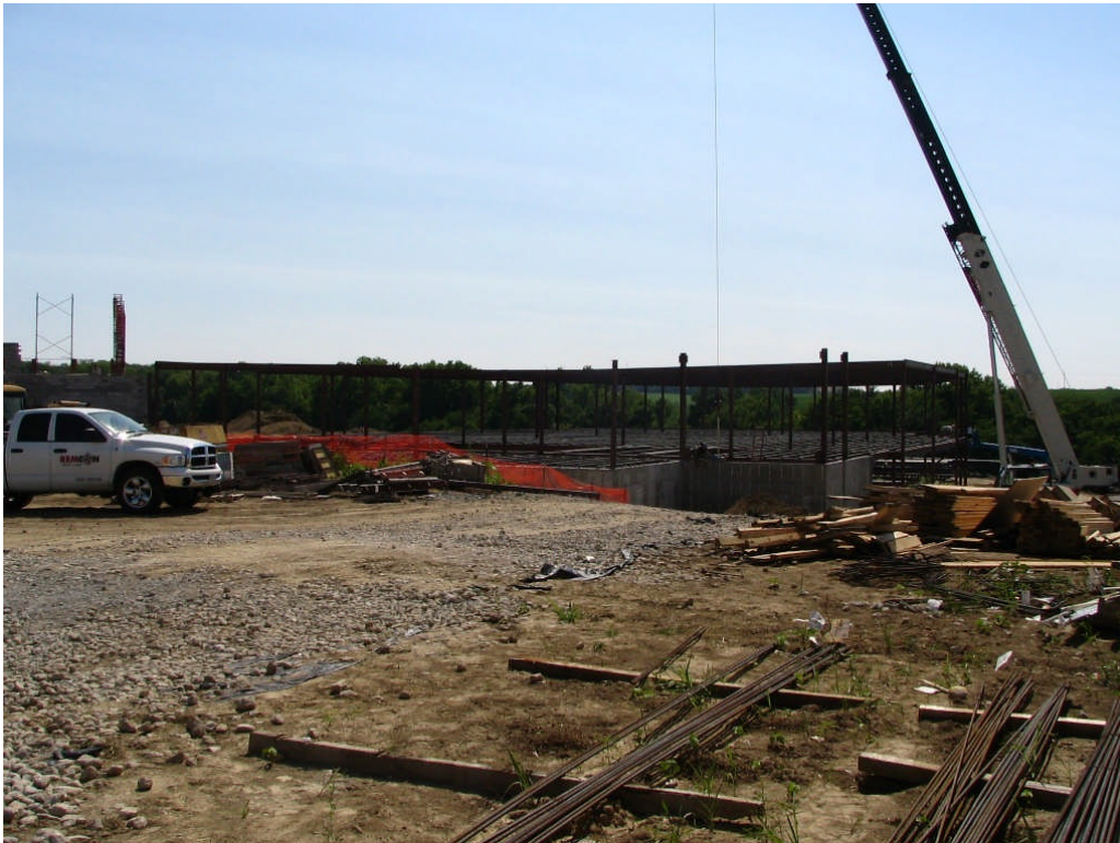
Elementary #24 – Steel Erection at Classrooms (July 5, 2006)
