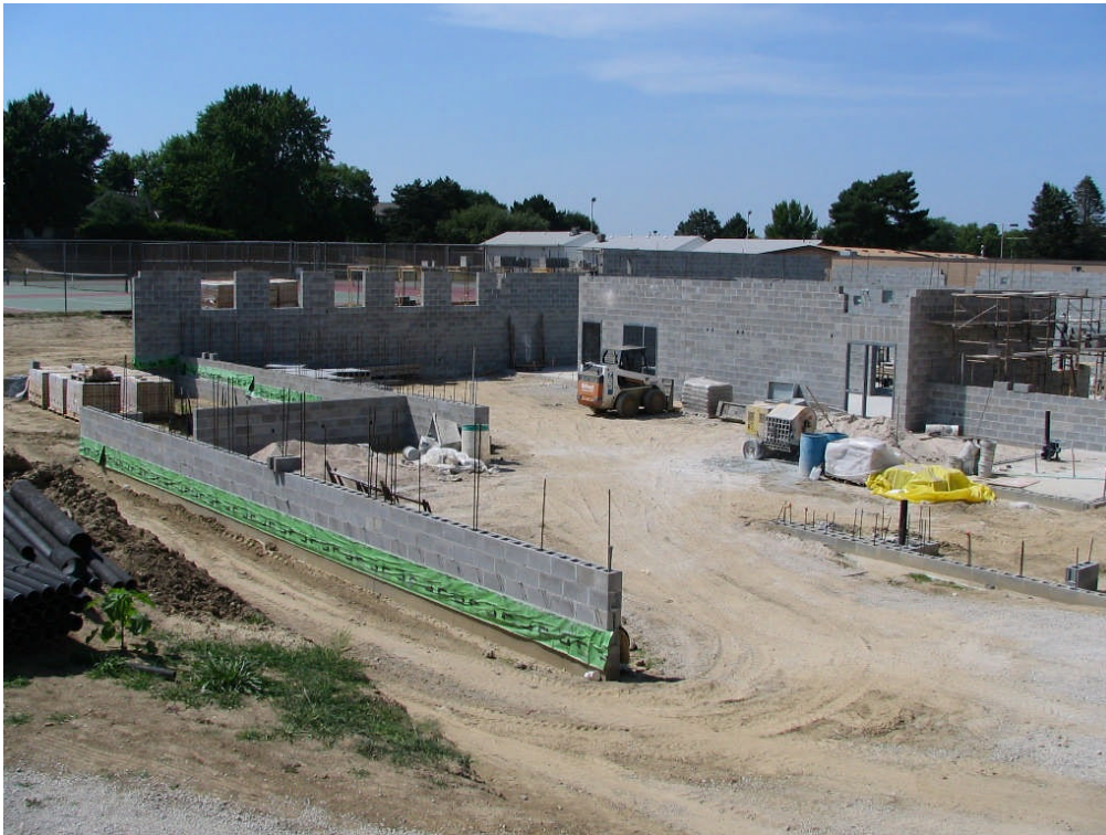
South High School – Building Addition (July 5, 2006)
