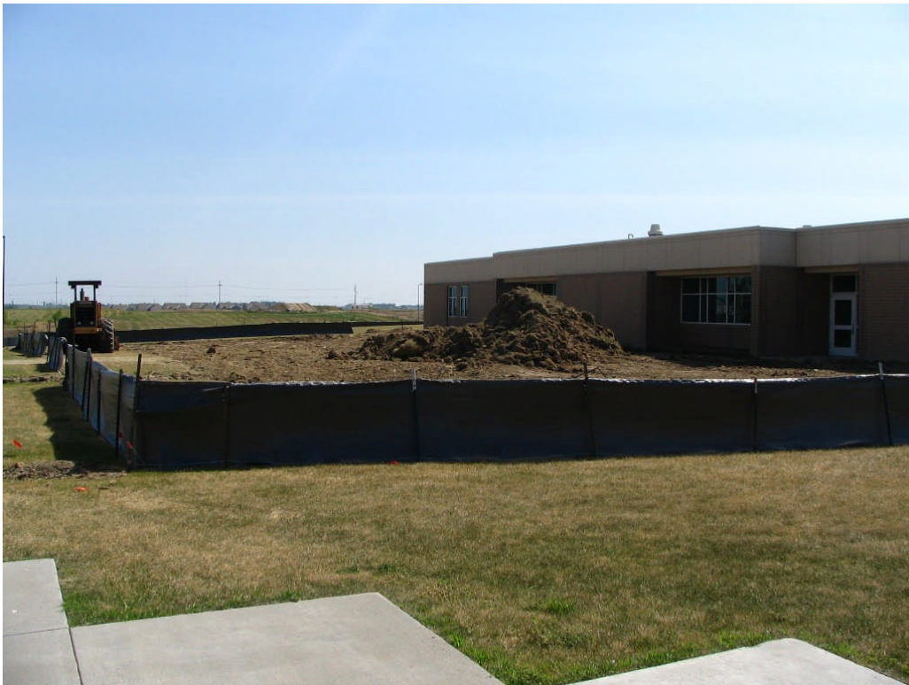
Beadle Middle School – Southwest Addition (July 5, 2006)
