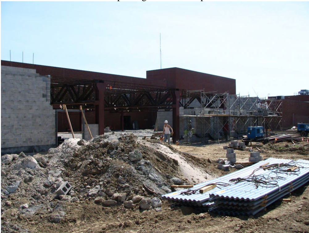
North High School – Building Addition (July 5, 2006)
