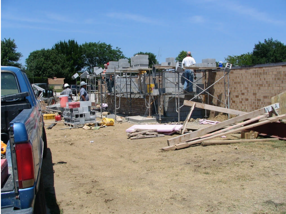
Ackerman Elementary – Exterior Masonry (July 5, 2006)
