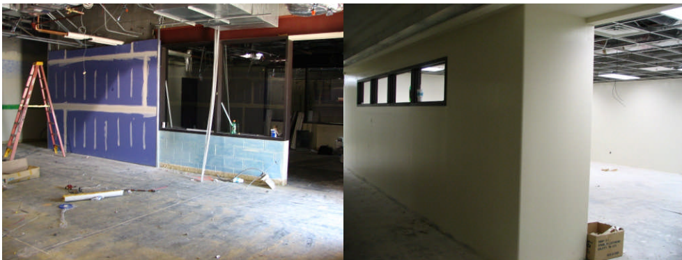
Ackerman Elementary – Interior Demolition and New Construction (July 5, 2006)
