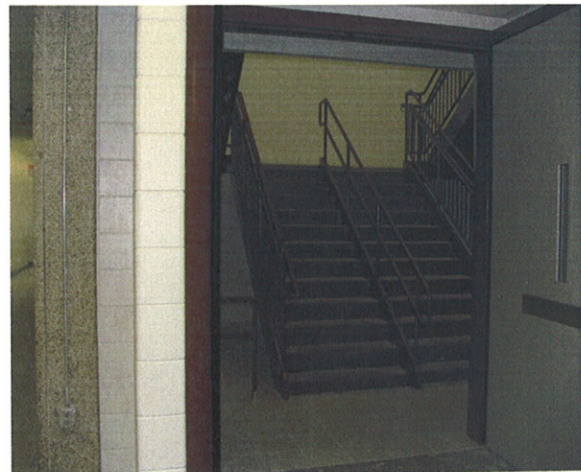
South High School - Quarry Tile missing at treads and risers of new stairwell (7/31/2006)
