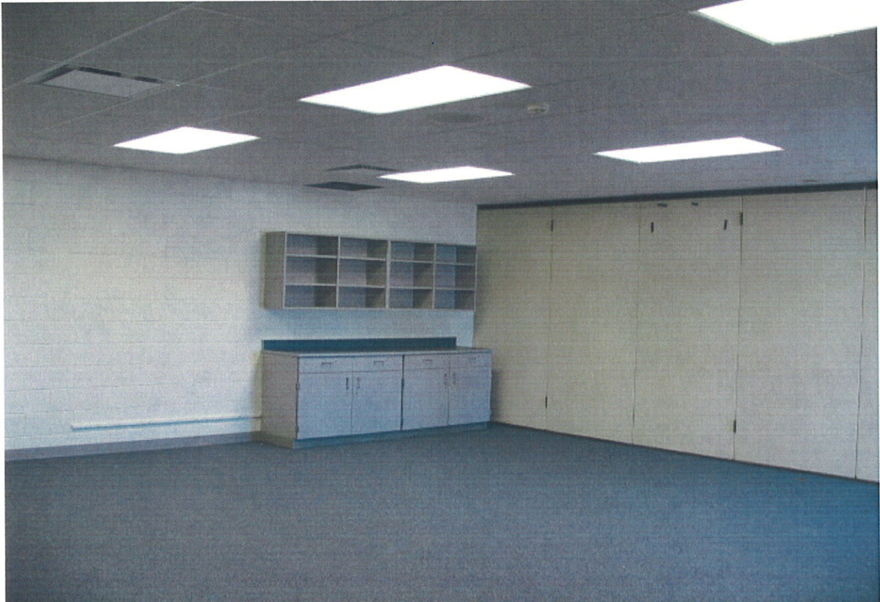
North High School - Typical classroom (7/31/2006)
