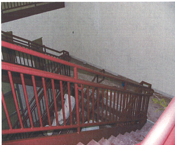
South High School - Quarry Tile missing at treads and risers of new stairwell (7/31/2006)
