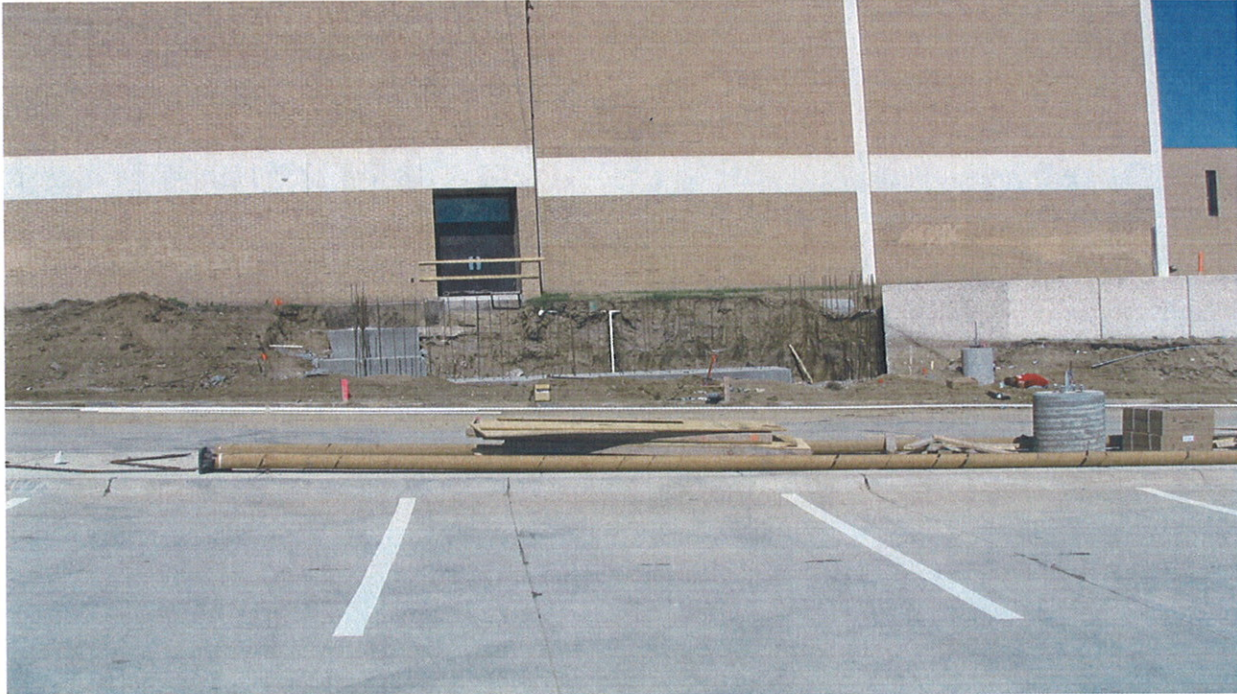
South High School - Retaining Wall (7/31/2006)
