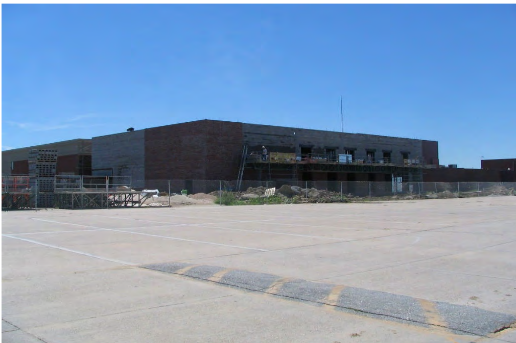
North High School – Building Addition (August 14, 2006)
