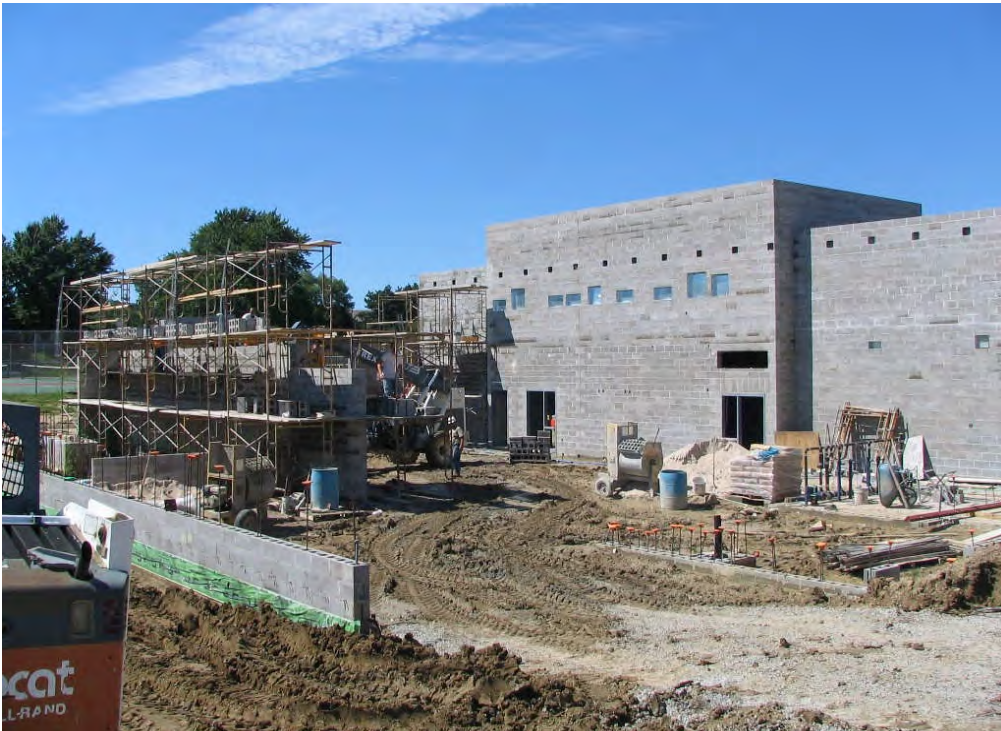
South High School – Building Addition (August 14, 2006)
