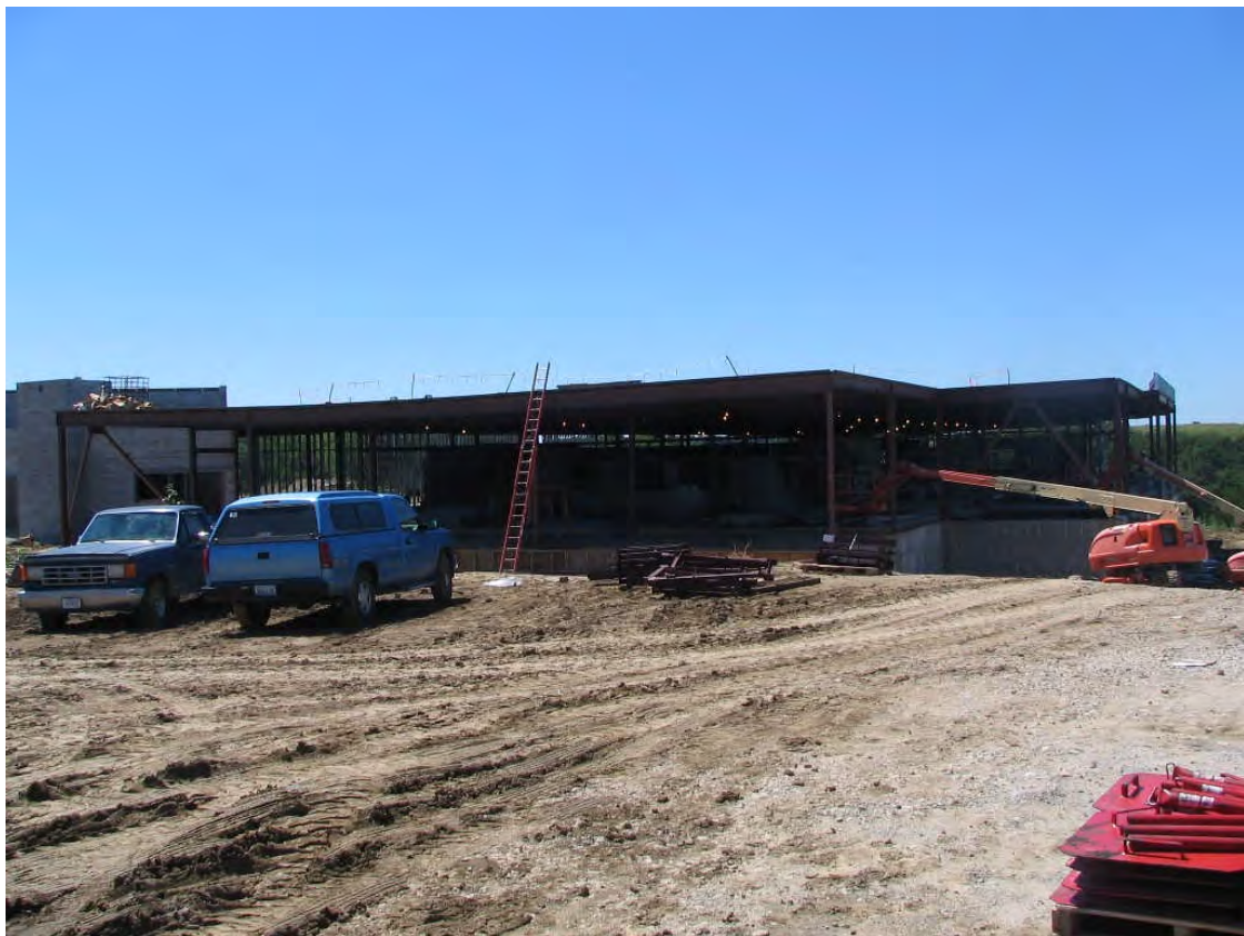
Elementary #24 – Interior wall construction @ classrooms (August 14, 2006)
