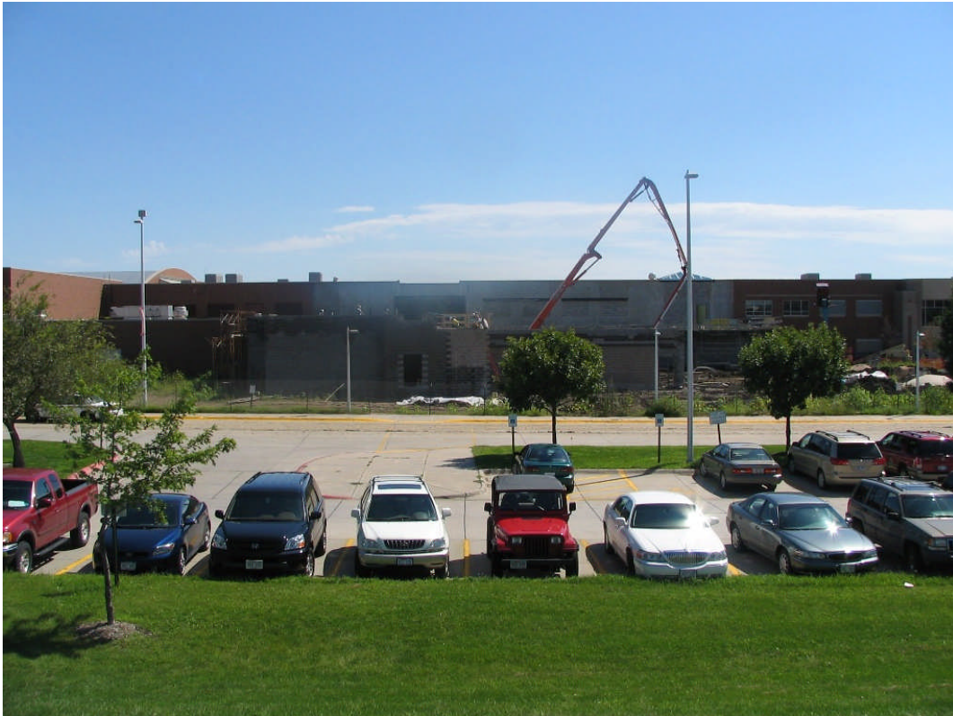
West High School – West Building Addition (August 29, 2006)
