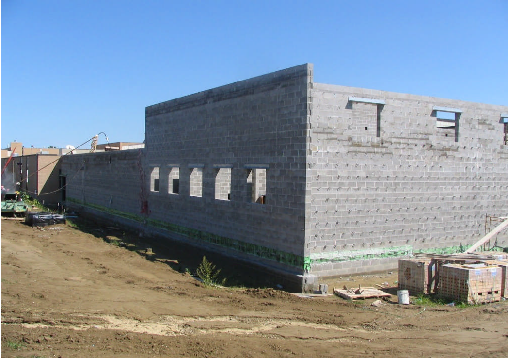
South High School – West Elevation Building Addition (August 29, 2006)
