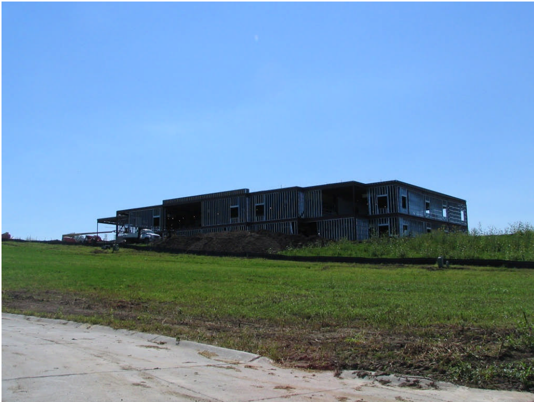
Elementary #24 – North Elevation (August 29, 2006)
