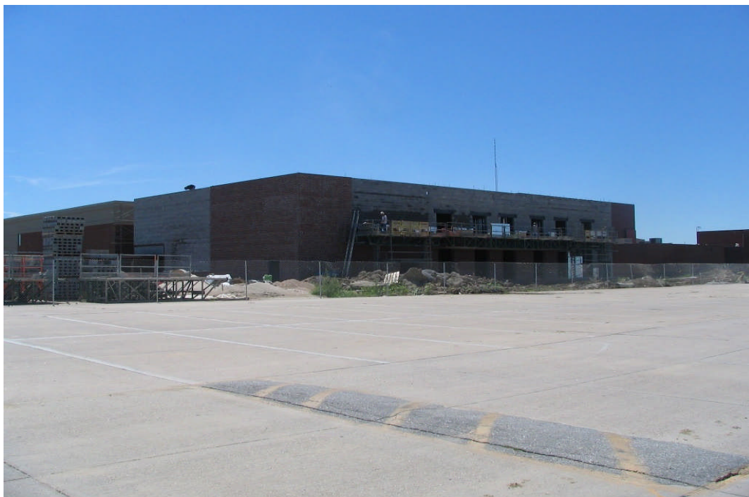
North High School – Building Addition (August 14, 2006)
