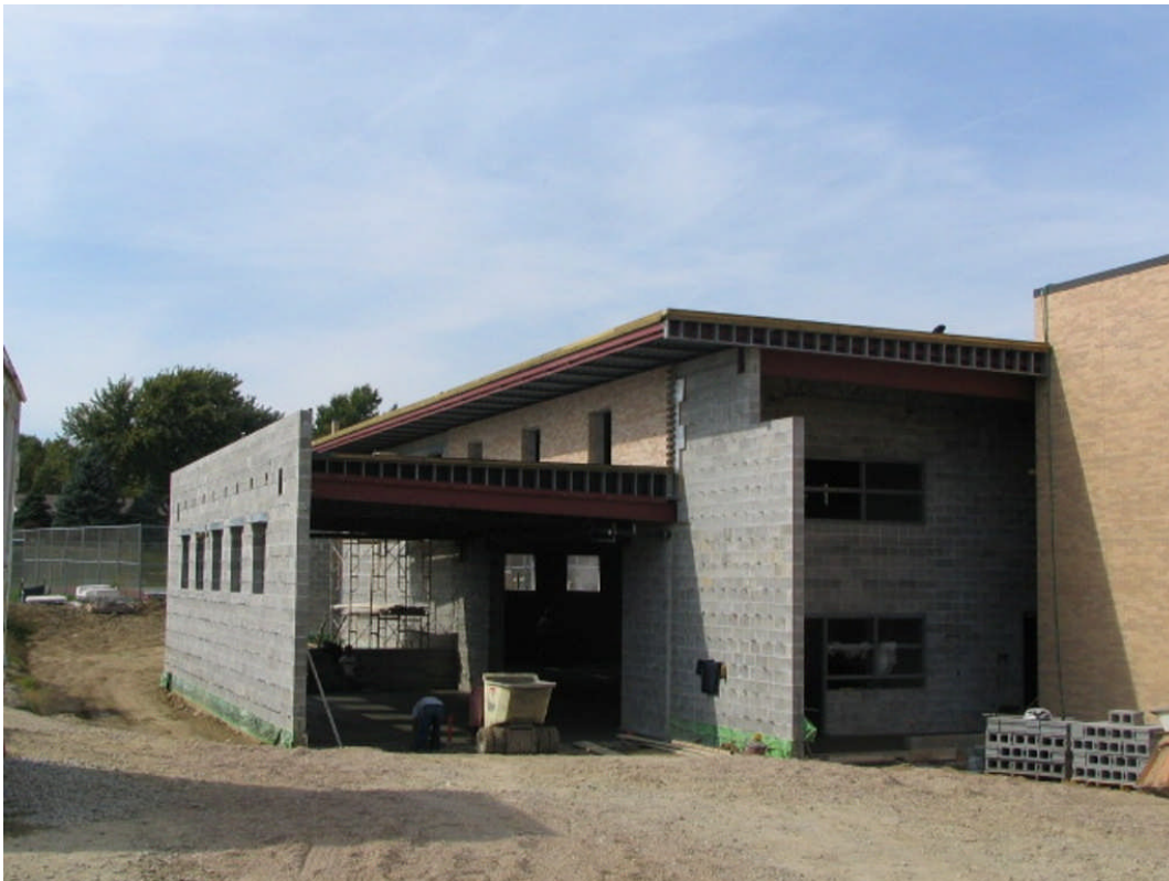
South High School – East Elevation Building Addition (October 6, 2006)
