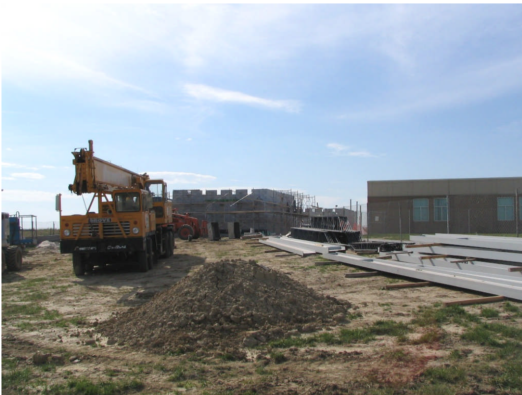
Beadle Middle School – South Building Addition (October 6, 2006)
