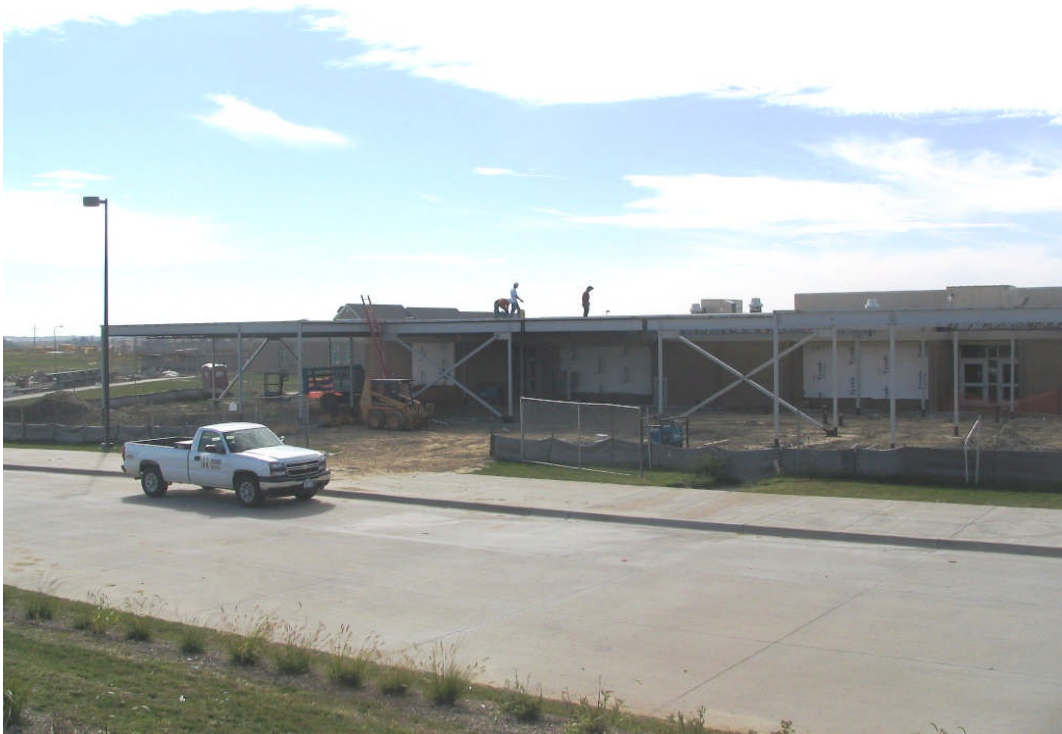
Beadle Middle School – East Building Addition (October 6, 2006)
