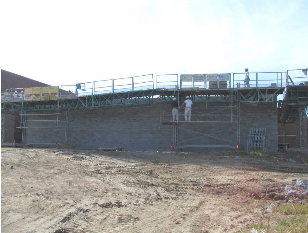
West High School – Band (east) Addition (October 6, 2006)
