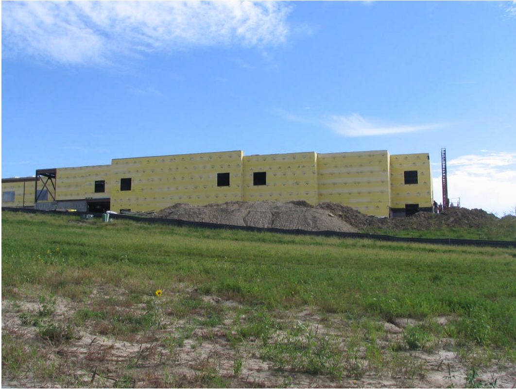
Elementary #24 – North Elevation (October 6, 2006)
