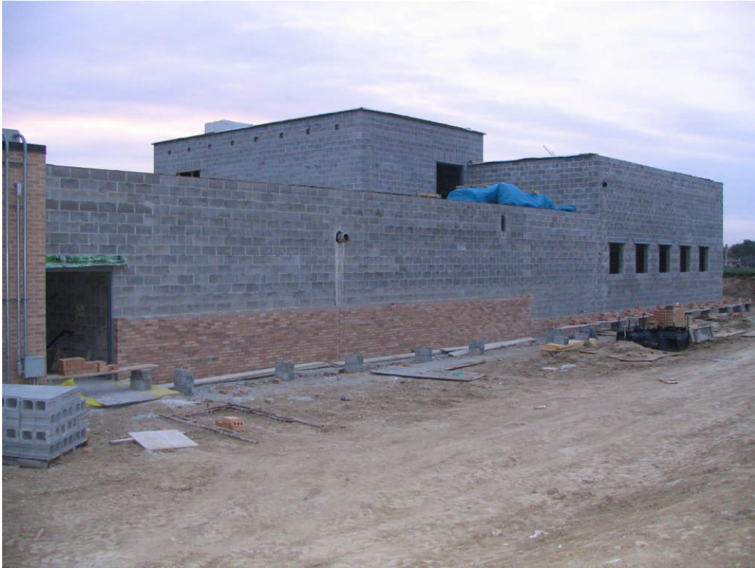
South High School – West Elevation Building Addition (October 09, 2006)
