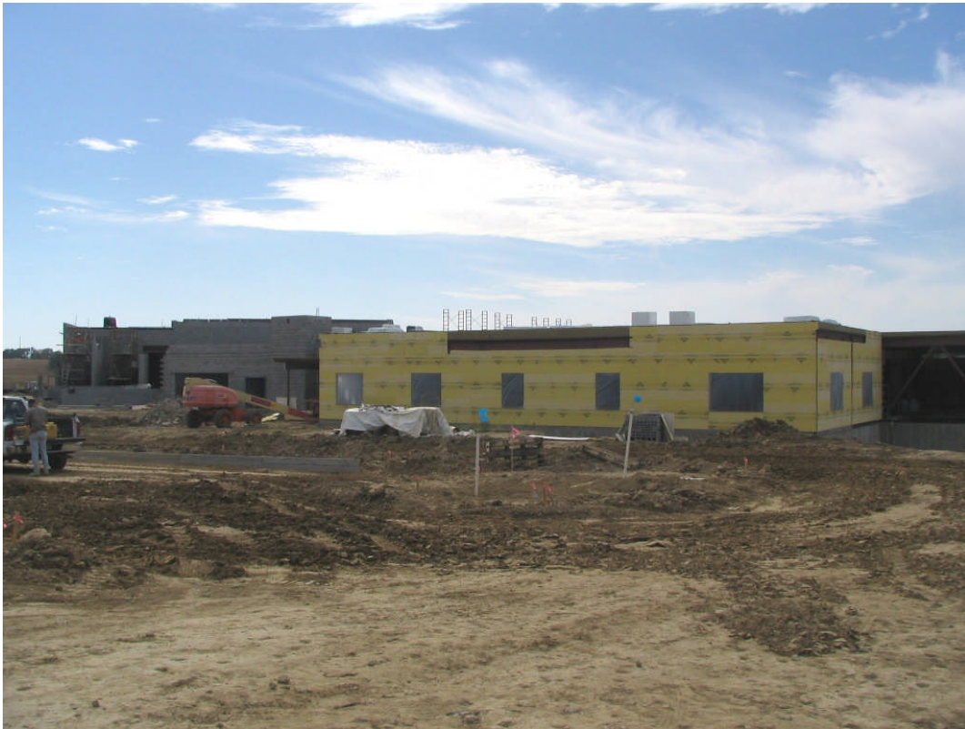
Elementary #24 – East Elevation (October 6, 2006)
