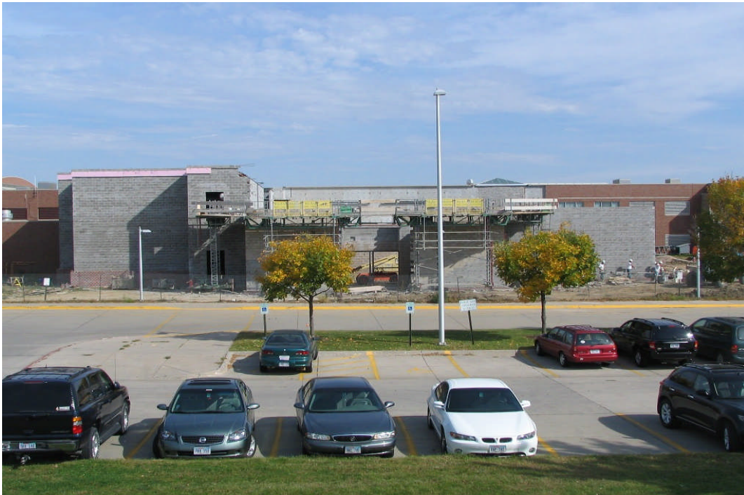
West High School – Classroom (west) Addition (October 6, 2006)
