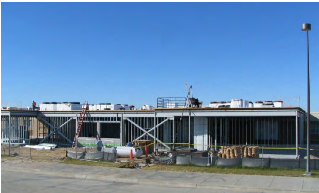
Beadle Middle School – East Building Addition (November 11, 2006)
