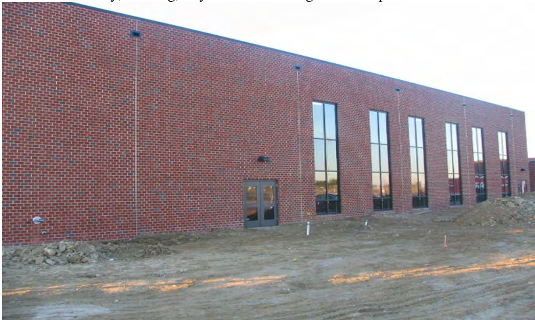
North High School – West Elevation Building Addition (November 13, 2006)
