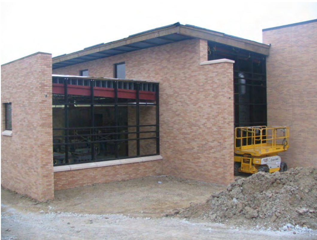
South High School – East Elevation Building Addition (November 13, 2006)
