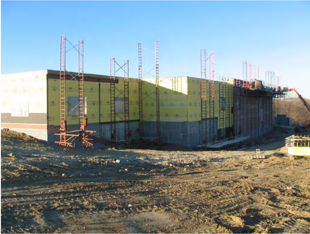
Elementary #24 – North Elevation (November 11, 2006)
