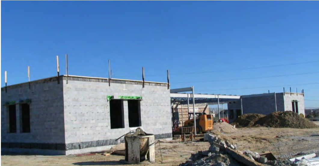
Beadle Middle School – South Building Addition (November 11, 2006)
