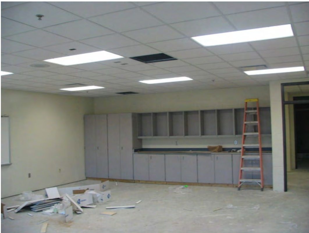
North High School – Typical Classroom Addition (November 13, 2006)
