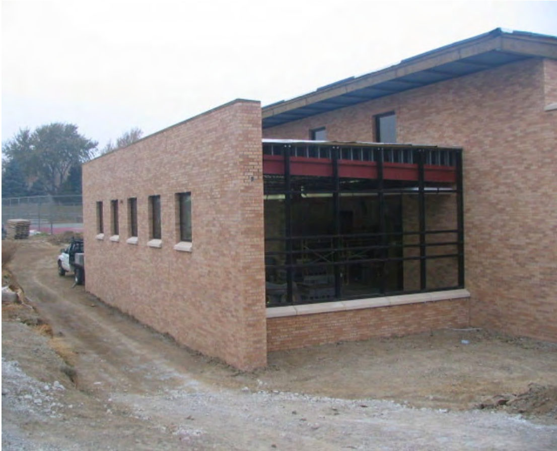
South High School – South Elevation Building Addition (November 13, 2006)
