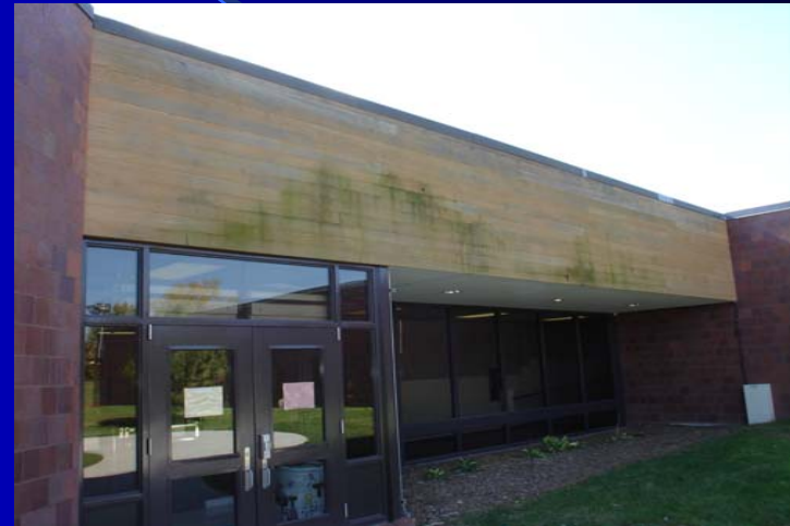
North Playground Entrance
