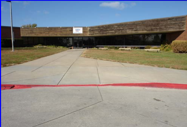
South Front Entrance
