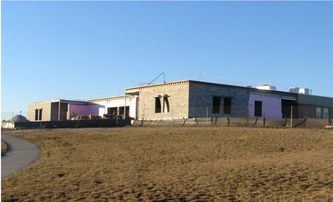
Beadle Middle School – South Building Addition (December 09, 2006)
