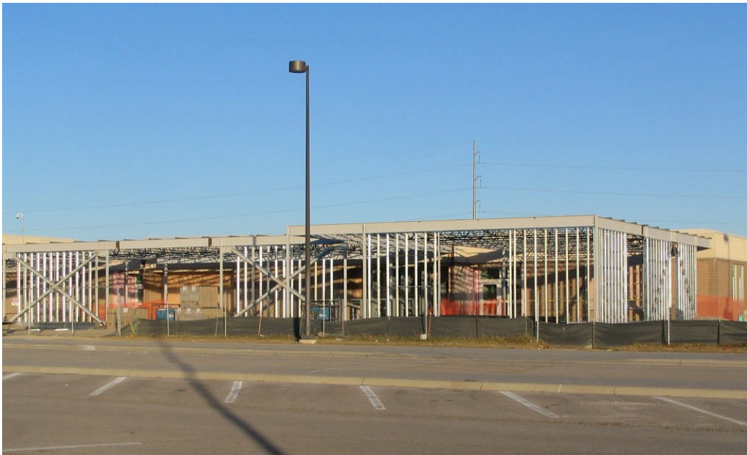
Beadle Middle School – West Building Addition (December 09, 2006)
