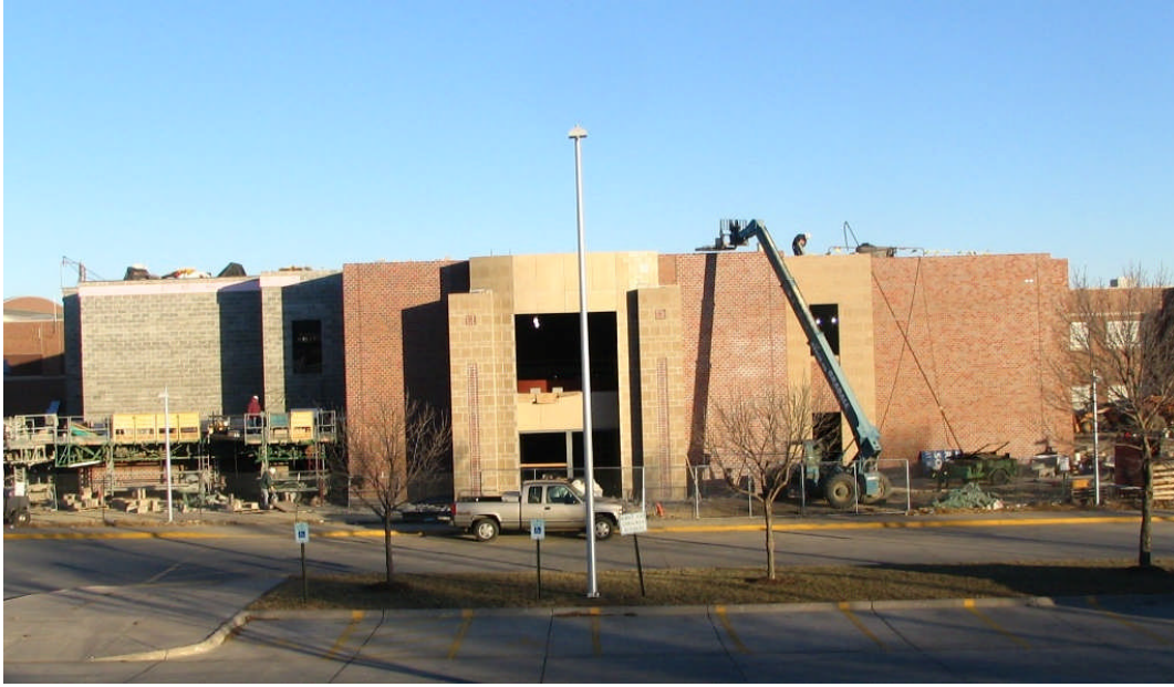
West High School – West Building Addition (December 09, 2006)
