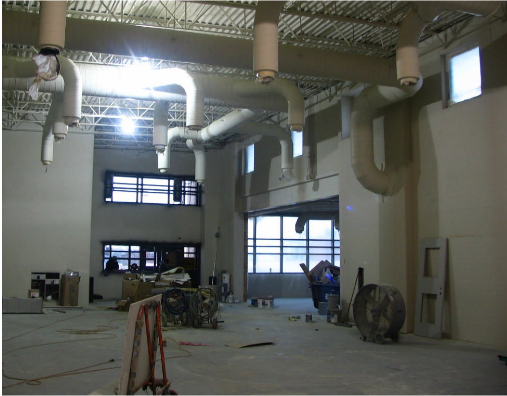
South High School – Fitness Interior Construction (December 11, 2006)
