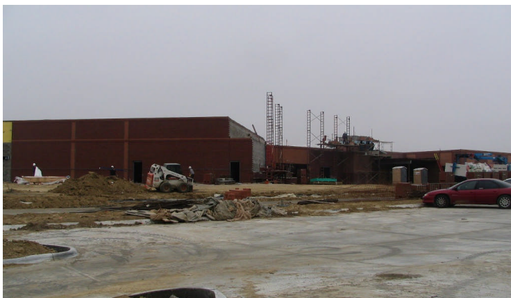
Elementary #24 – East Elevation (December 11, 2006)
