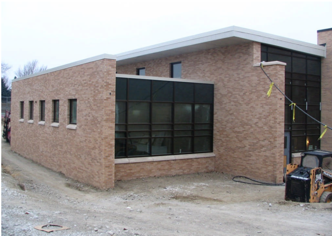
South High School – East Entrance (December 11, 2006)
