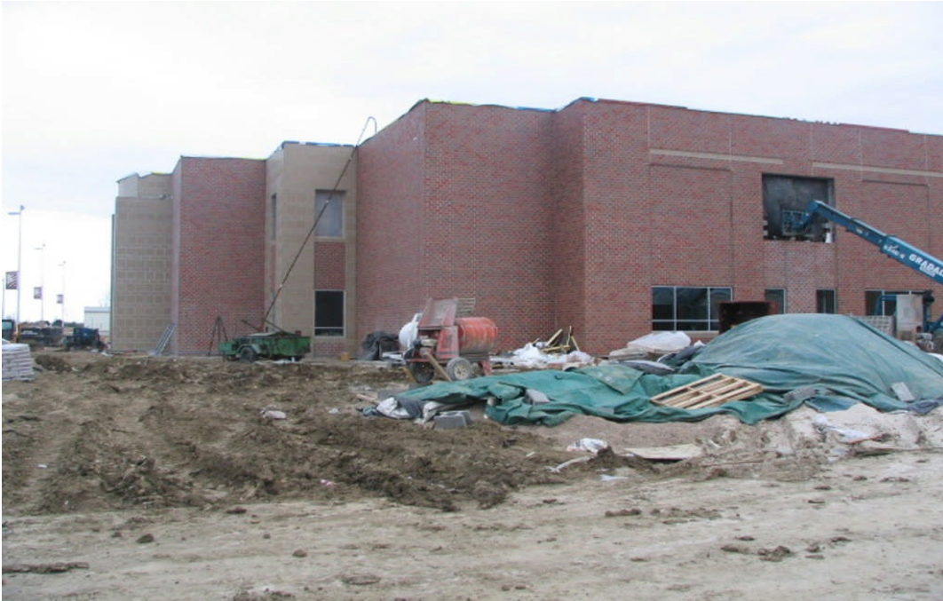
West High School – West Building Addition (January 11, 2007)
