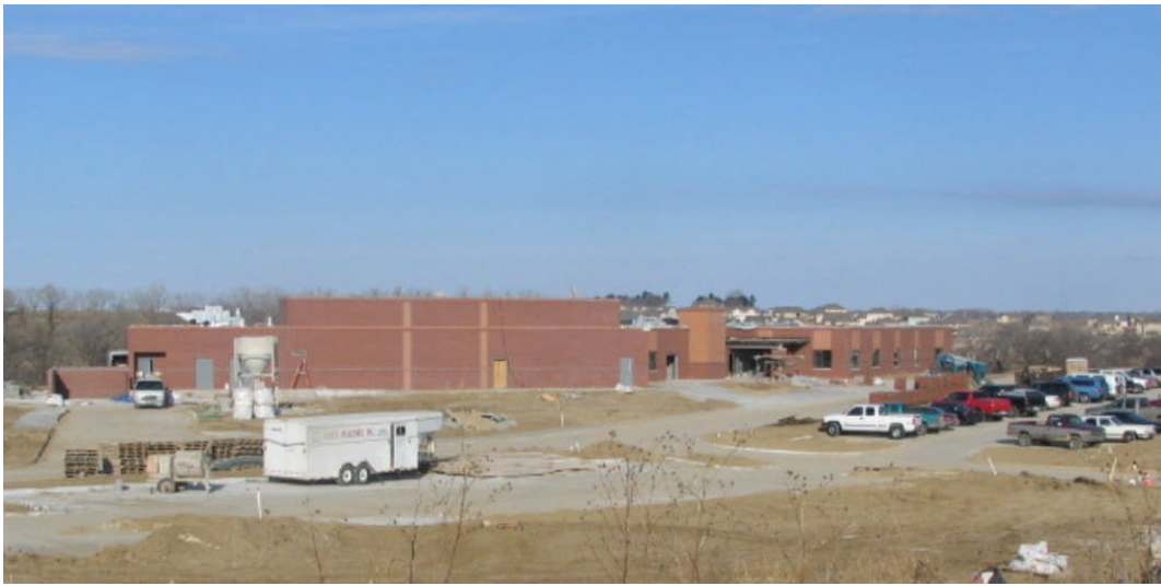
Reagan Elementary #24 – East Elevation (January 11, 2007)
