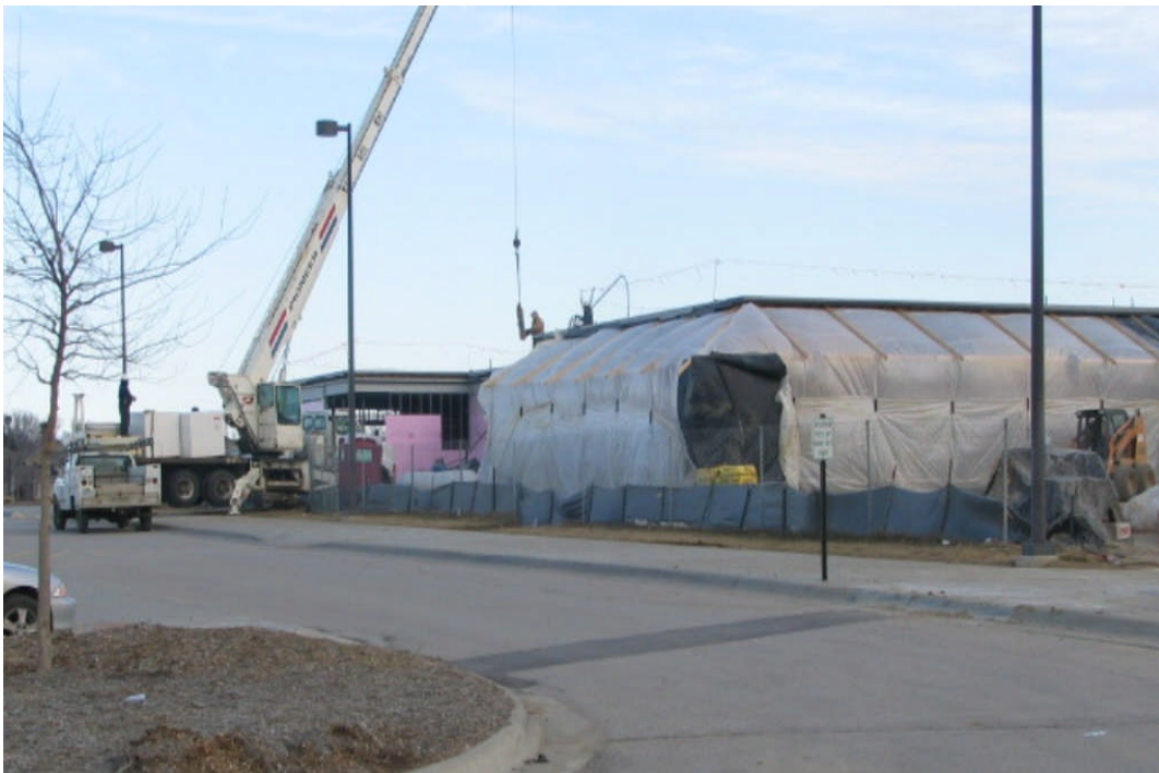
Beadle Middle School – West Building Addition (January 11, 2007)
