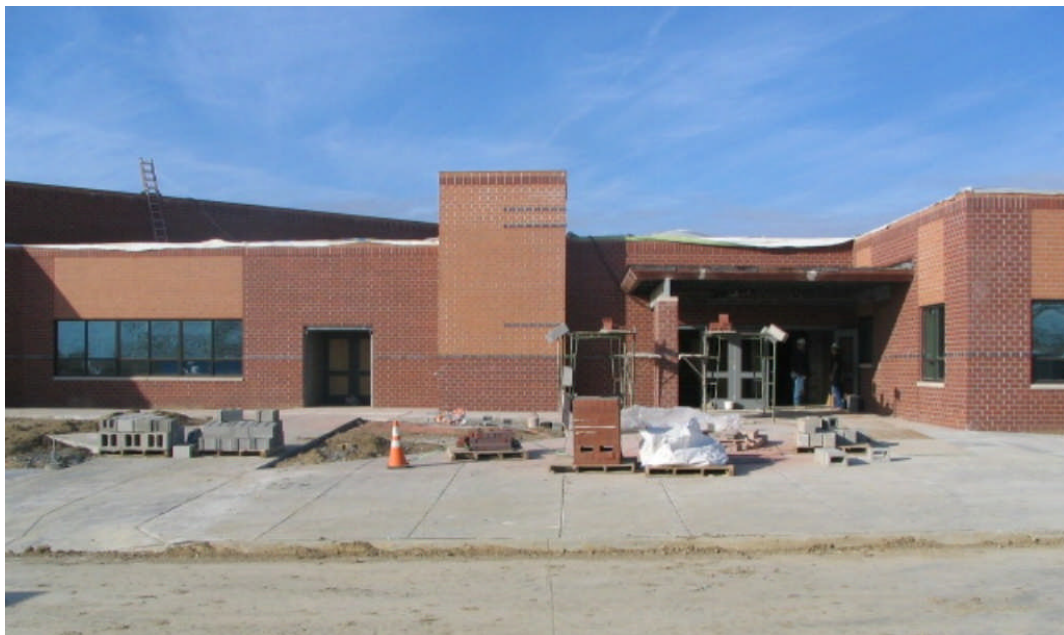
Reagan Elementary #24 – Entry Elevation (January 11, 2007)
