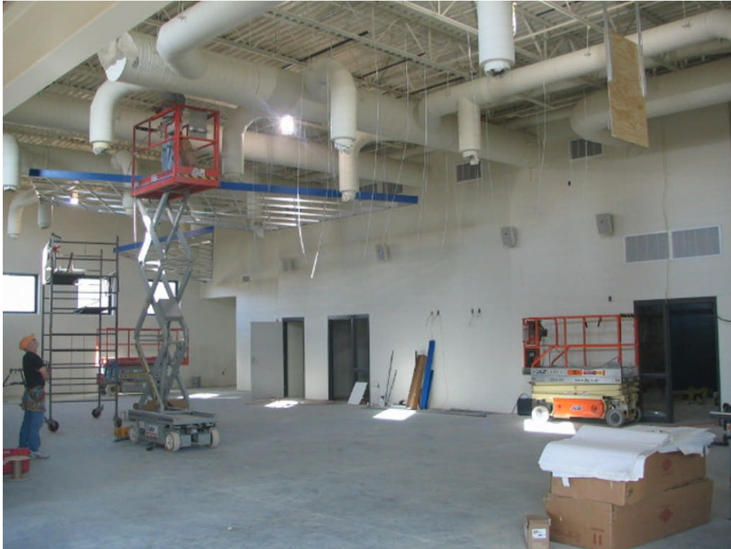
South High School – Fitness Interior Construction (January 11, 2007)
