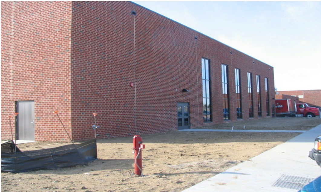
North High School – North Elevation Building Addition (January 11, 2007)
