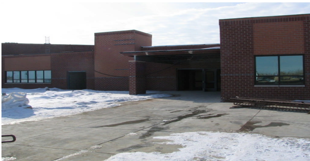
Reagan Elementary #24 – Entry Elevation (February 09, 2007)
