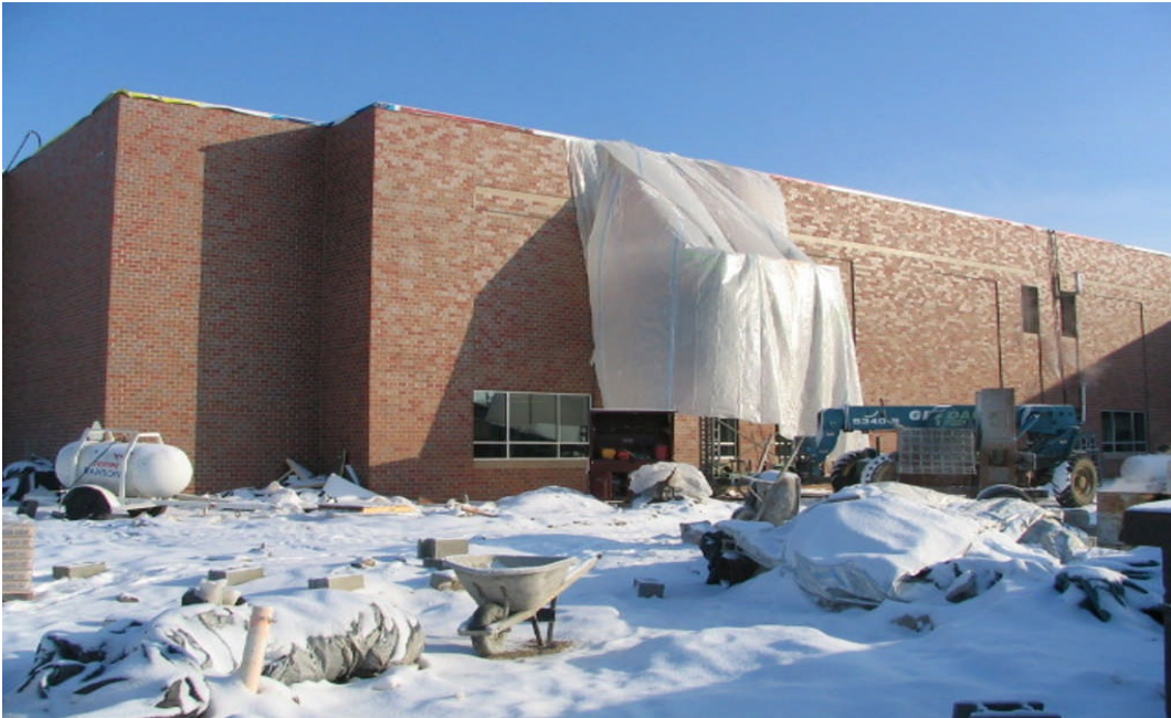
West High School – West Building Addition (February 08, 2007)
