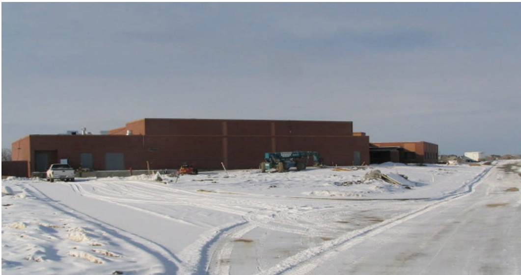
Reagan Elementary #24 – East Elevation (February 09, 2007)
