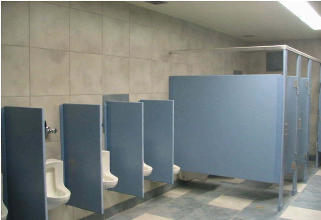
North High School – Restroom Replacement (February 12, 2007)
