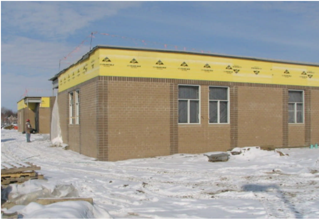
Beadle Middle School – West Wing Addition (February 09, 2007)
