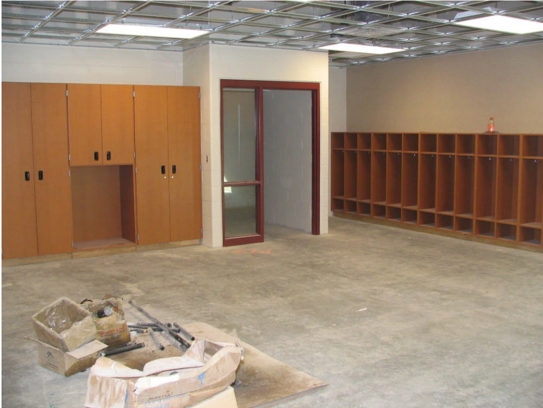
Reagan Elementary #24 – Typical Classroom (March 07, 2007)
