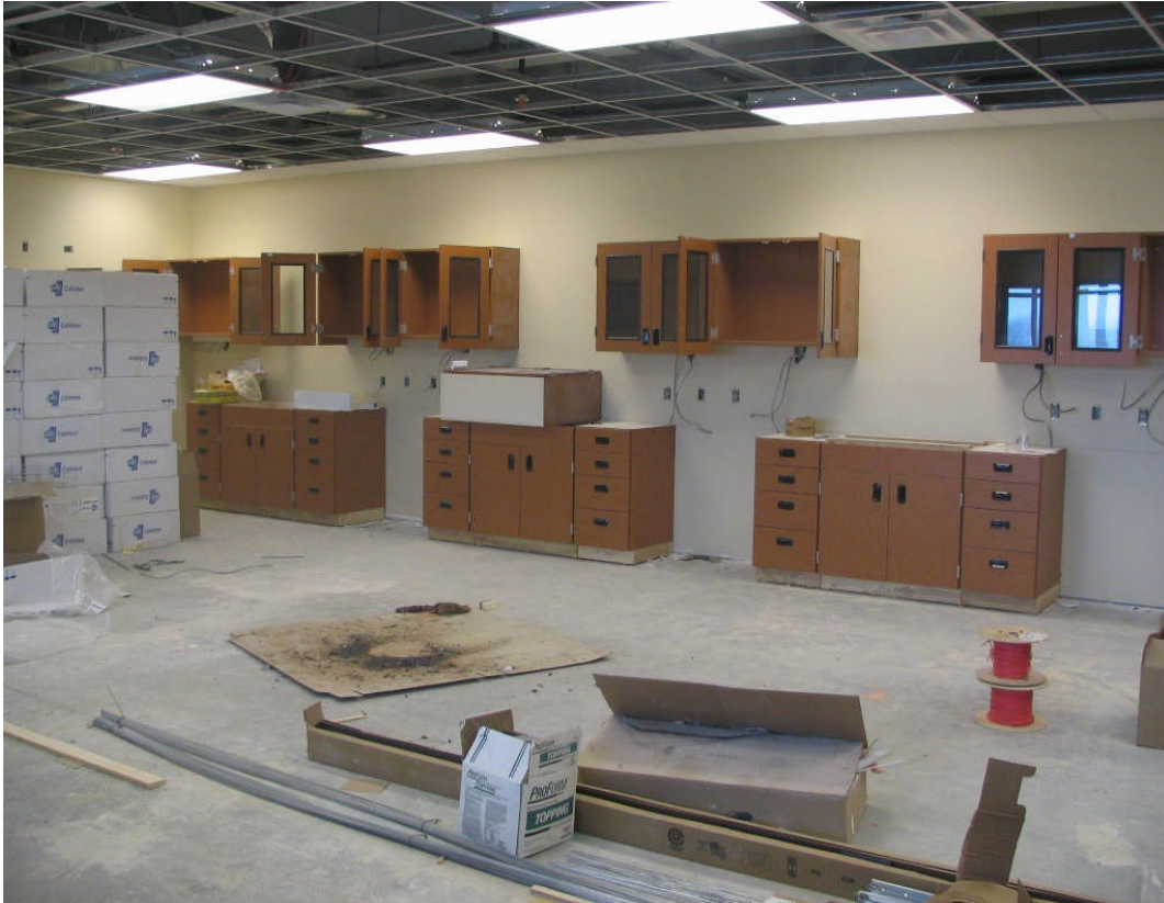
Beadle Middle School – East Wing Classroom (March 07, 2007)
