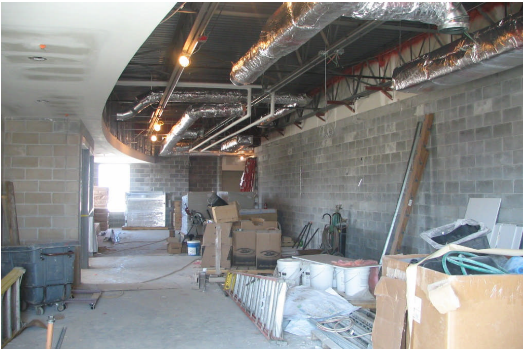
West High School – Classroom Addition - Upper Level Commons (March 12, 2007)
