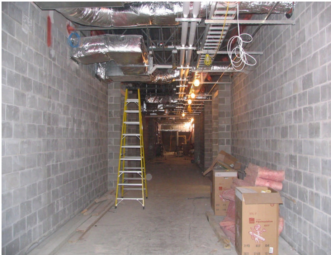
West High School – Classroom Addition - Upper Level Corridor (March 12, 2007)
