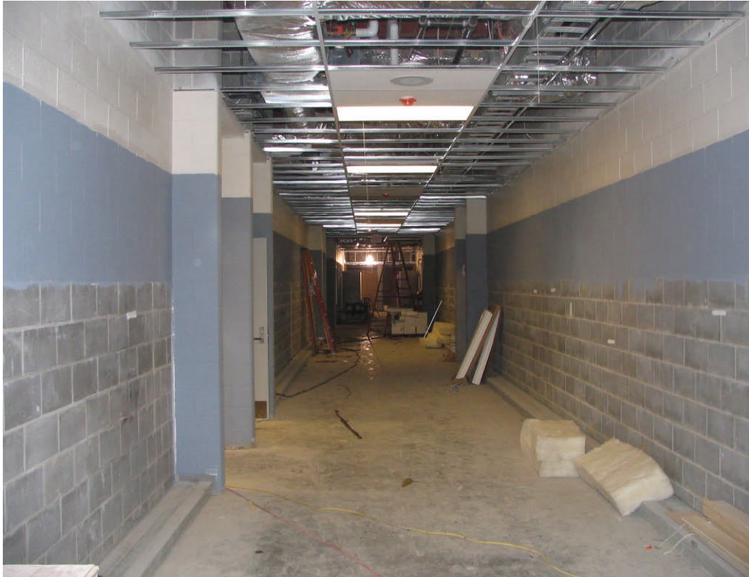
West High School – Classroom Addition - Lower Level Corridor (March 12, 2007)
