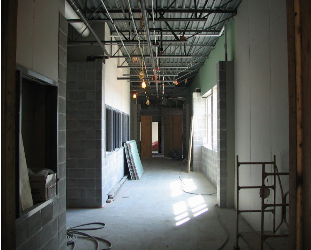
Beadle Middle School – West Wing Corridor (March 12, 2007)
