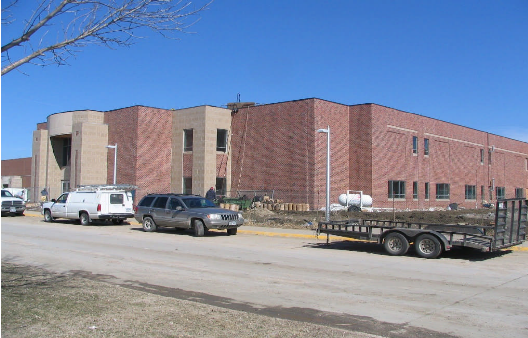
West High School – Classroom Addition (March 12, 2007)
