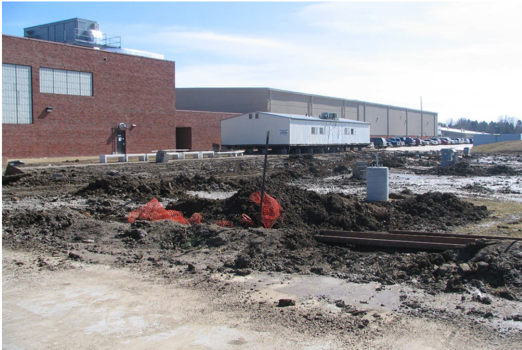
North High School – Portable Removal (March 12, 2007)
