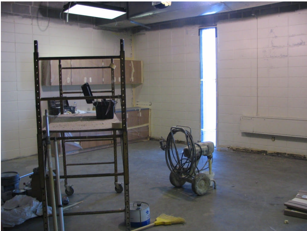
South High School – Typical Classroom Renovation (March 05, 2007)
