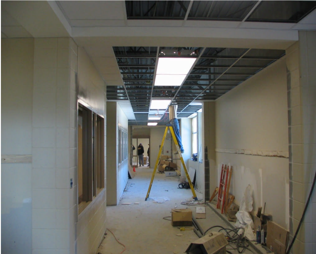
Beadle Middle School – East Wing Corridor (March 12, 2007)
