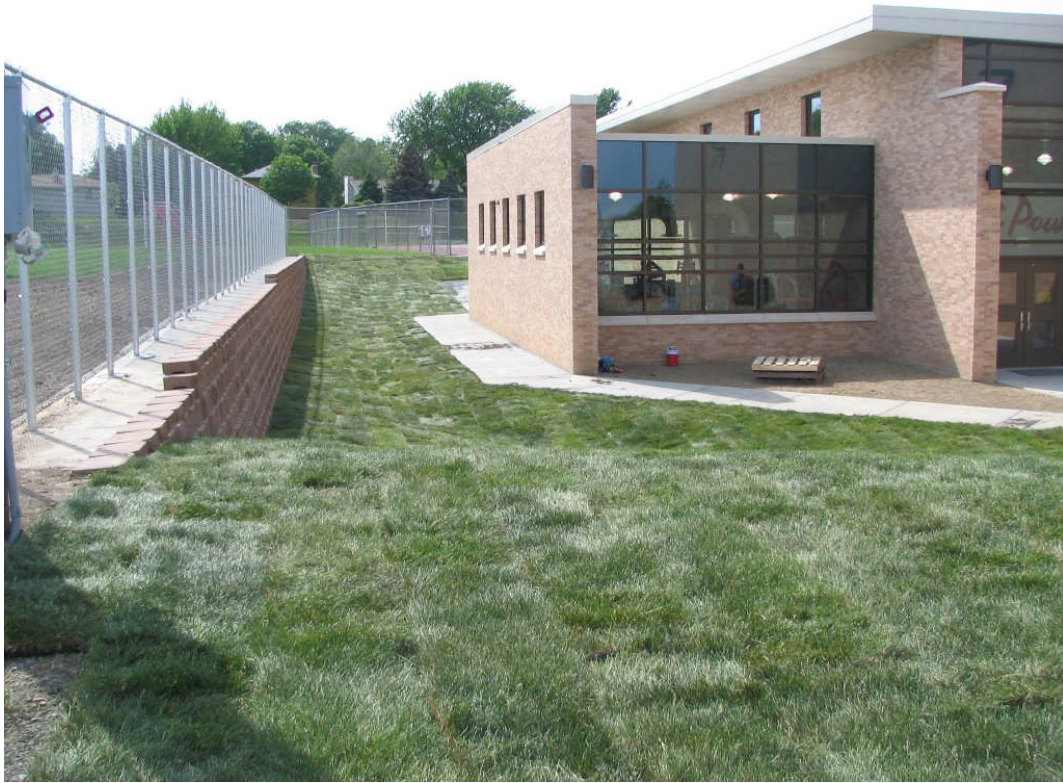
South High School – Exterior of Addition (May 14, 2007)
