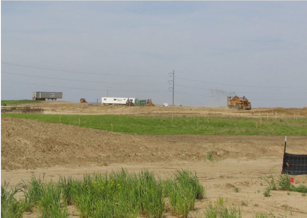
Upchurch Elementary #25 Earthmoving Operations (May 14, 2007)
