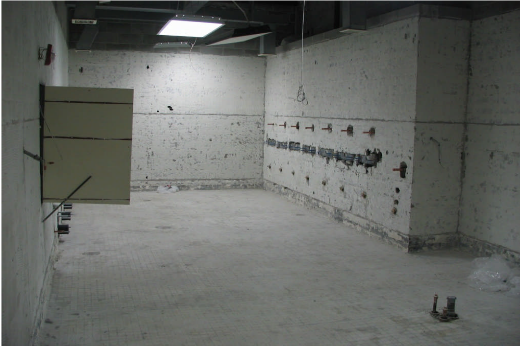
North High School – Restroom Renovations (May 14, 2007)
