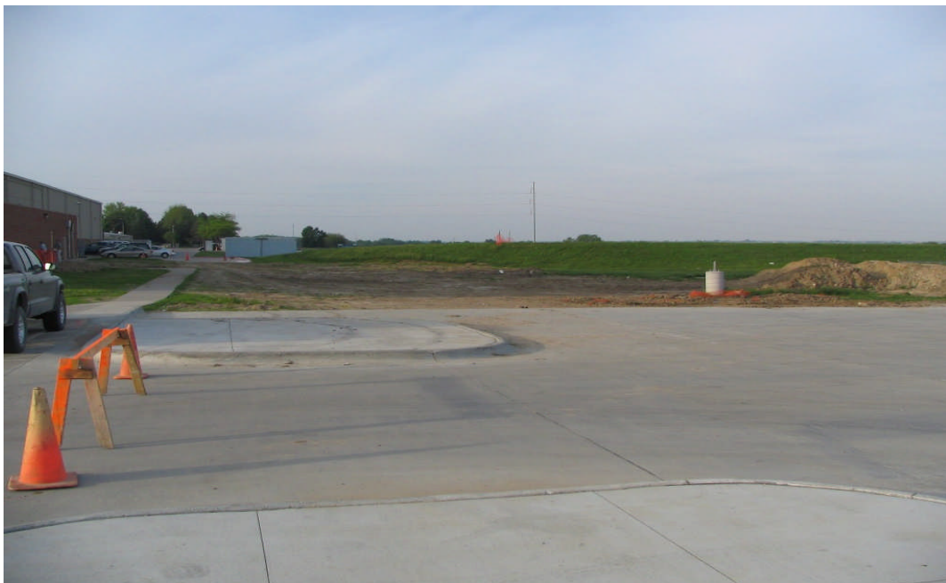
North High School – West side paving started (May 14, 2007)
