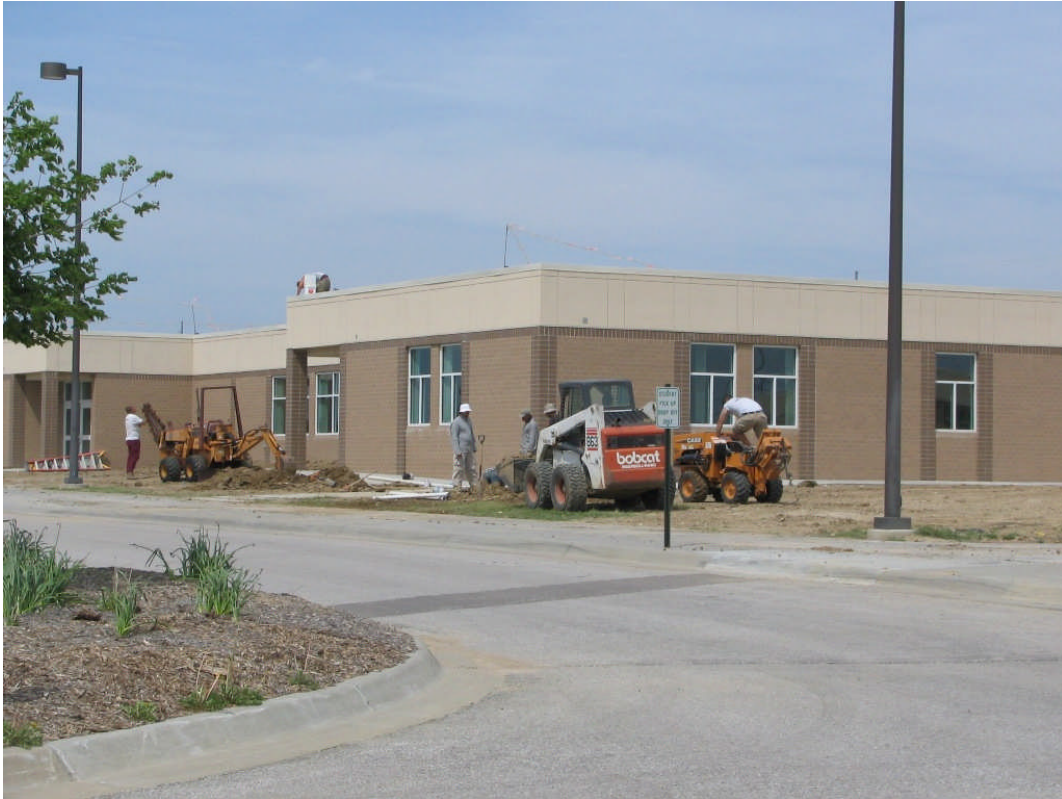
Beadle Middle School – West wing exterior irrigation work (May 14, 2007)
