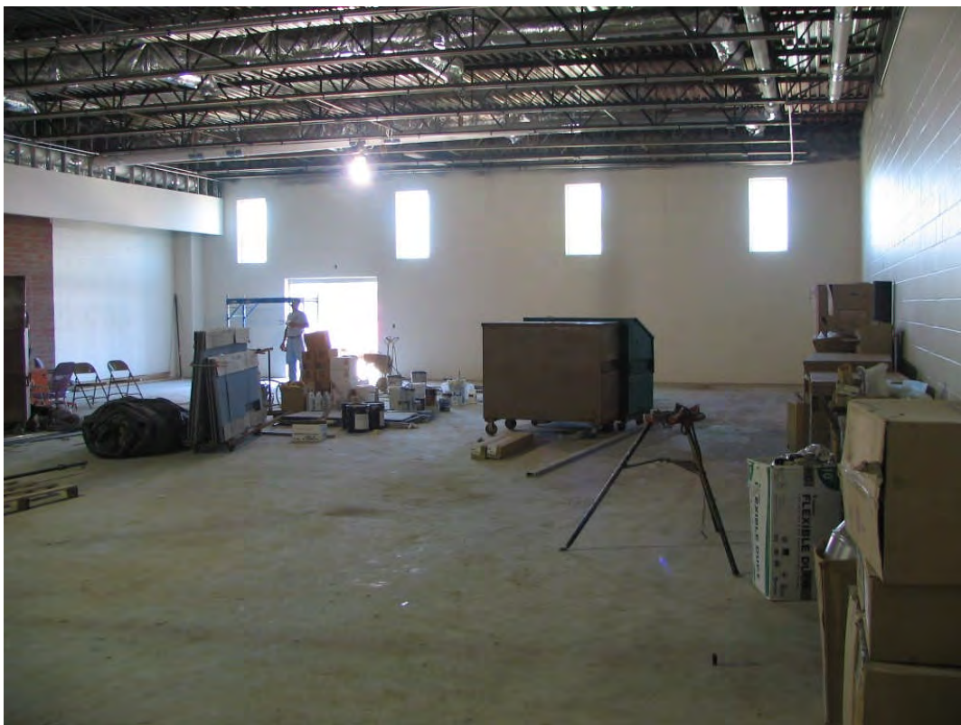
West High School – Band Room Addition (June 6, 2007)
