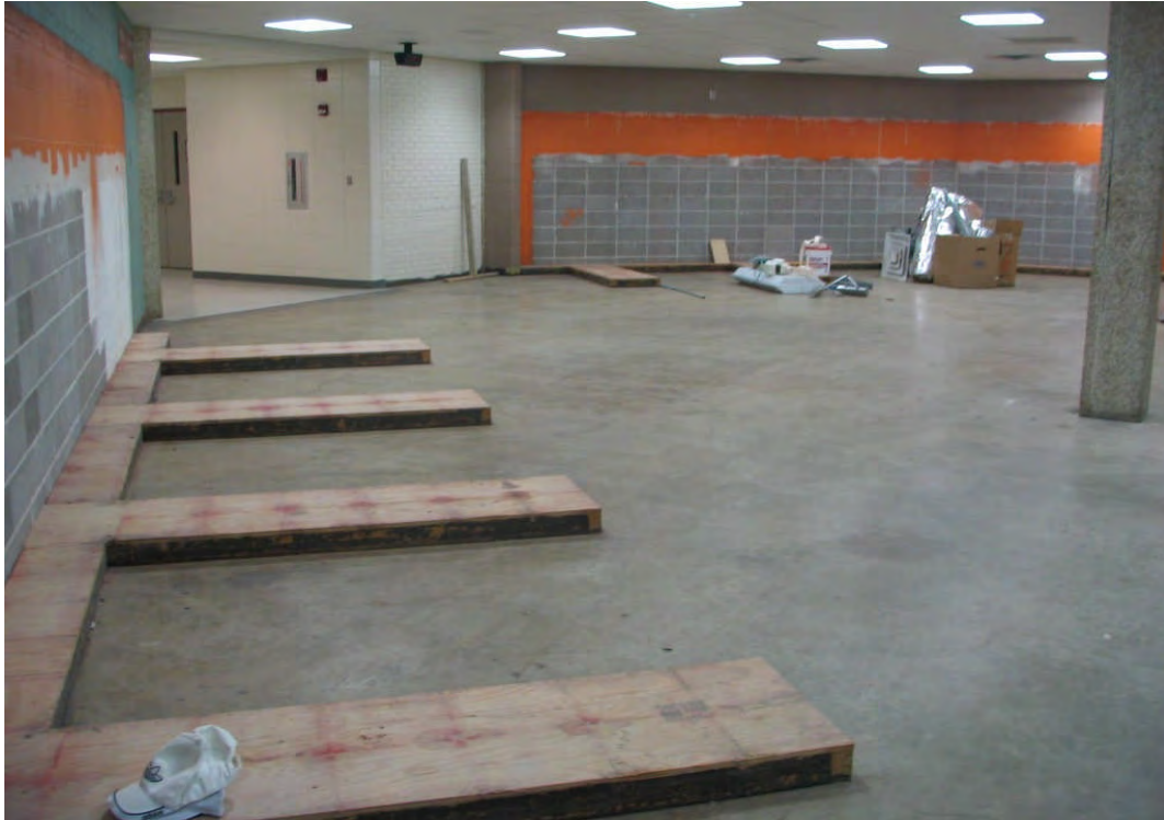
South High School – Stair renovation area (June 4, 2007)
