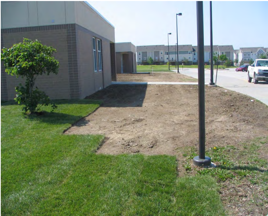
Beadle Middle School – West wing exterior sod work (June 4, 2007)
