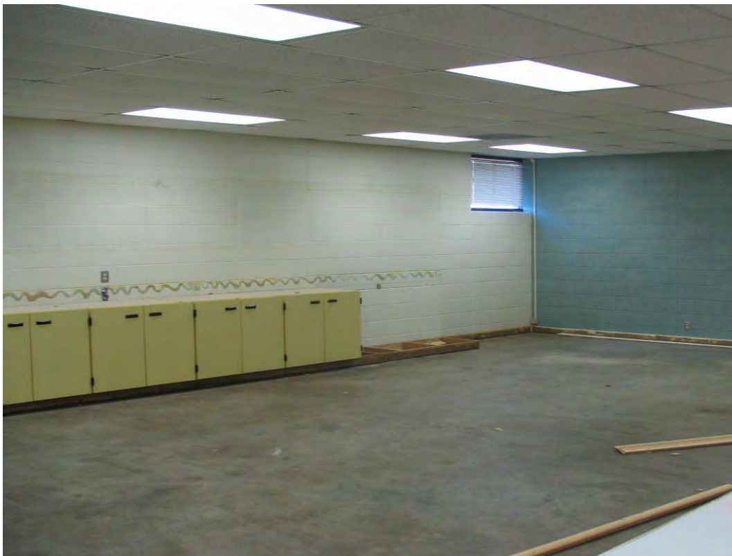
South High School – 300 wing renovations (June 4, 2007)
