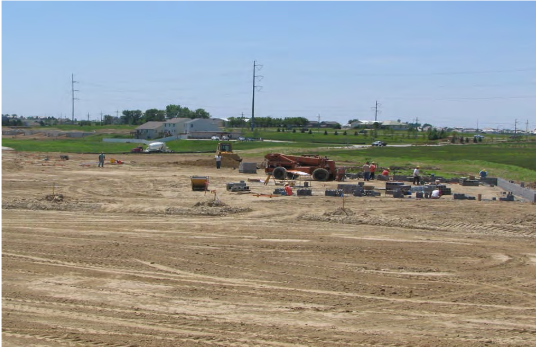
Upchurch Elementary #25 Foundation/ Masonry work started (June 6, 2007)
