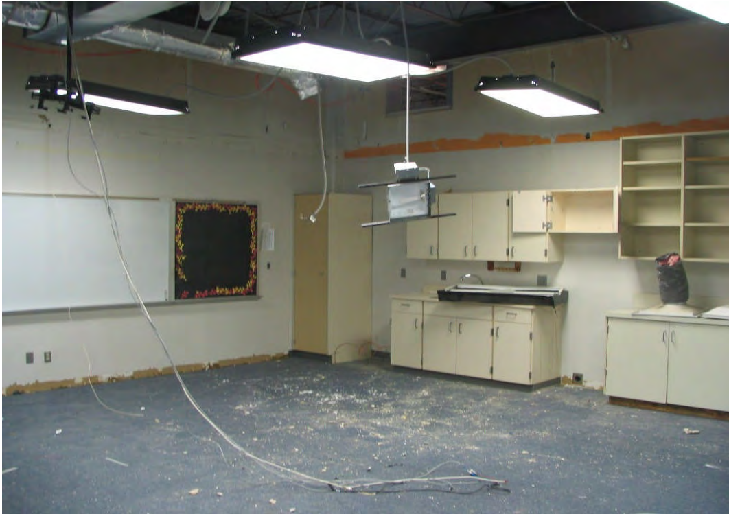
North High School – Classroom Renovations (June 6, 2007)
