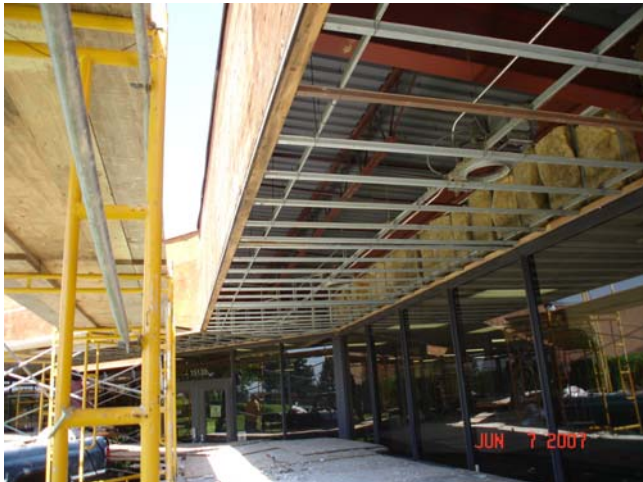
South Front Entrance
