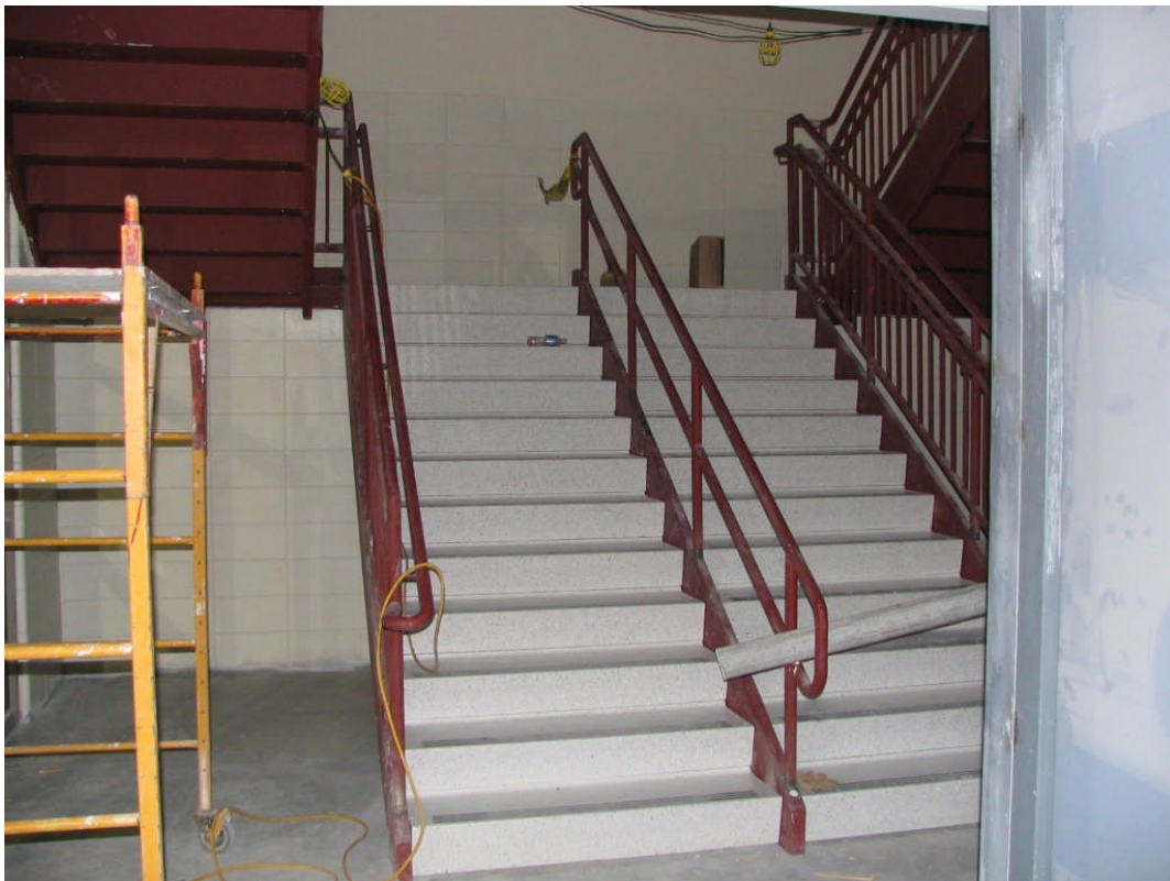
South High School – Stair Replacement (July 23, 2007)
