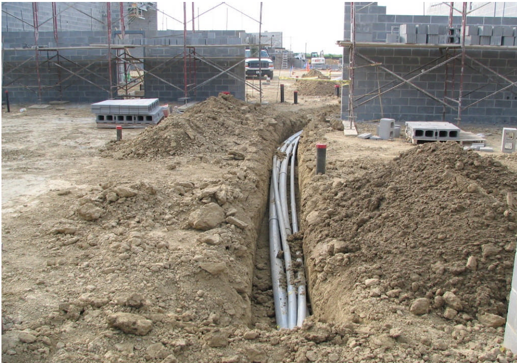
Upchurch Elementary #25 Electrical underground work in progress (July 24, 2007)
