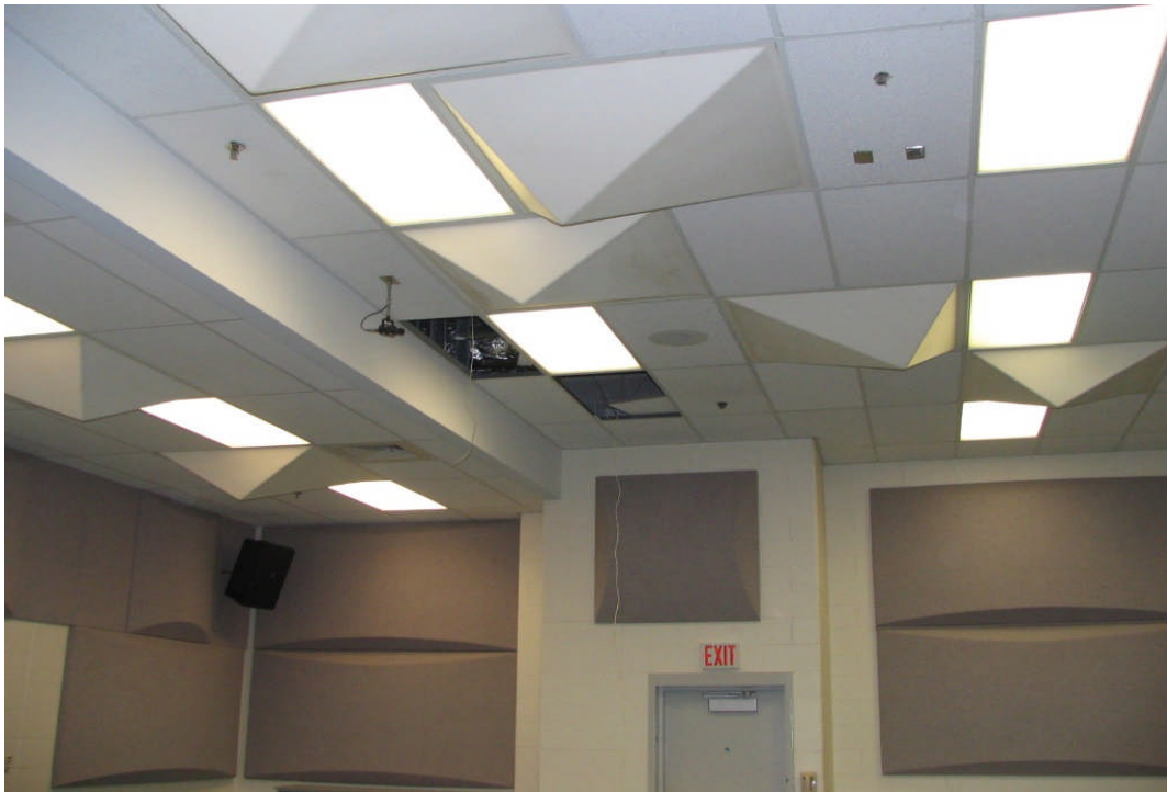
West High School – Coral Room Renovation (July 27, 2007)
