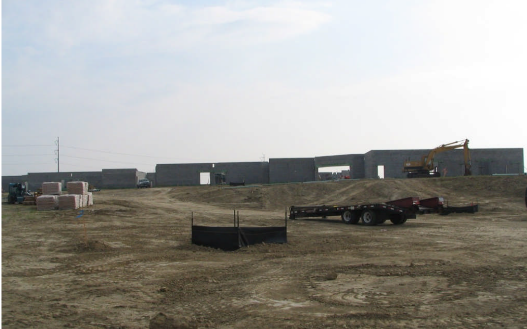
Upchurch Elementary #25 Foundation/ Masonry work in progress (July 24, 2007)
