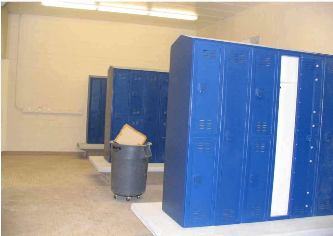
North High School – Locker Room Renovation (July 30, 2007)
