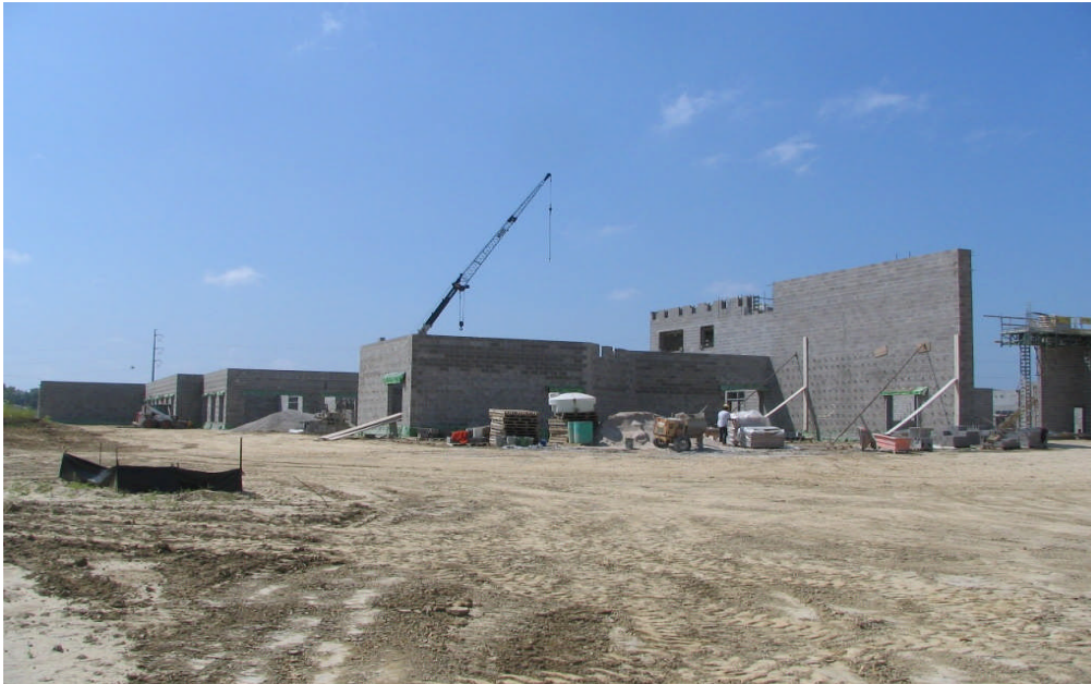
Upchurch Elementary #25 Masonry work in progress (Sept 6, 2007)
