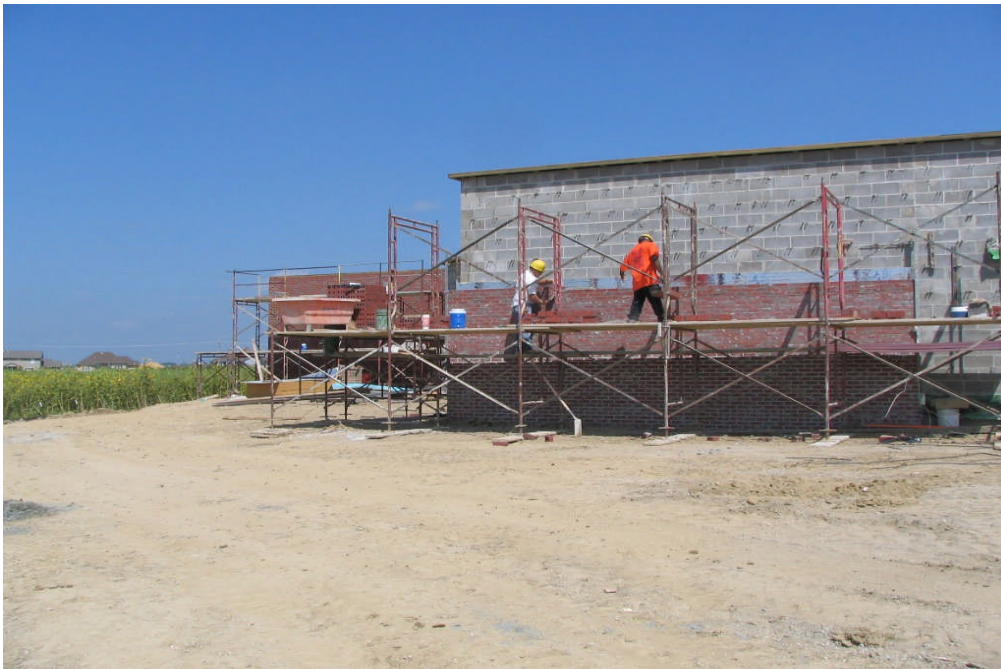
Upchurch Elementary #25 Brick work in progress (Sept 6, 2007)
