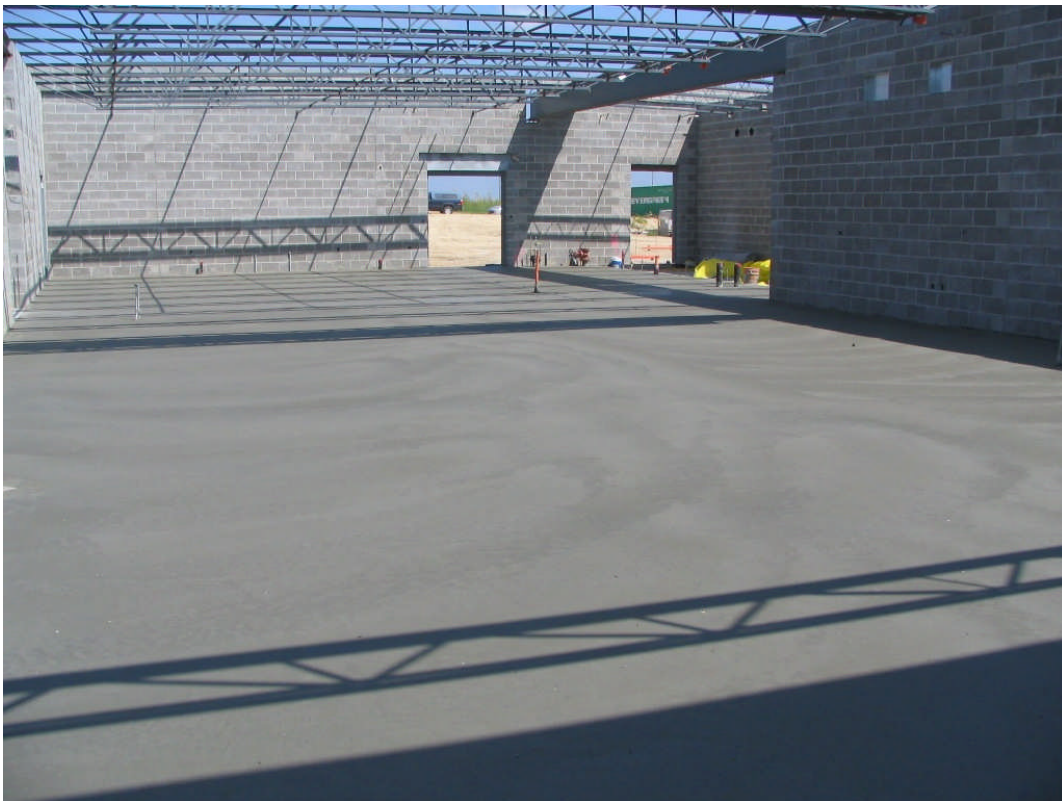
Upchurch Elementary #25 Concrete slab work started (Sept 6, 2007)
