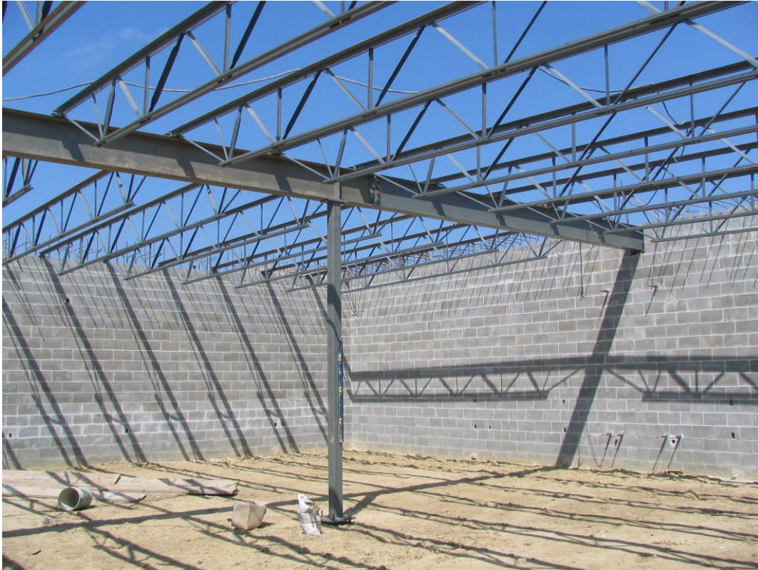
Upchurch Elementary #25 Structural Steel work in progress (Sept 6, 2007)
