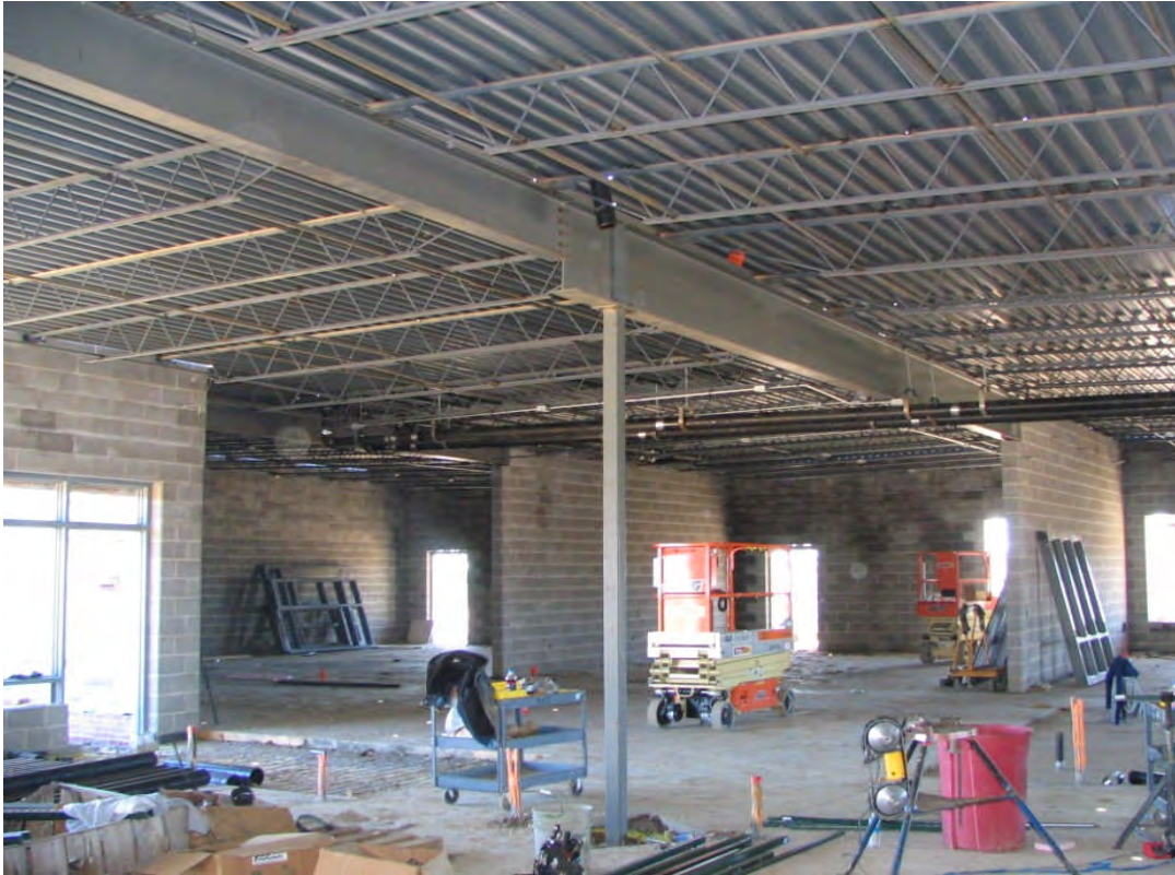
Upchurch Elementary #25 Interior mechanical installation underway (Oct 3, 2007)
