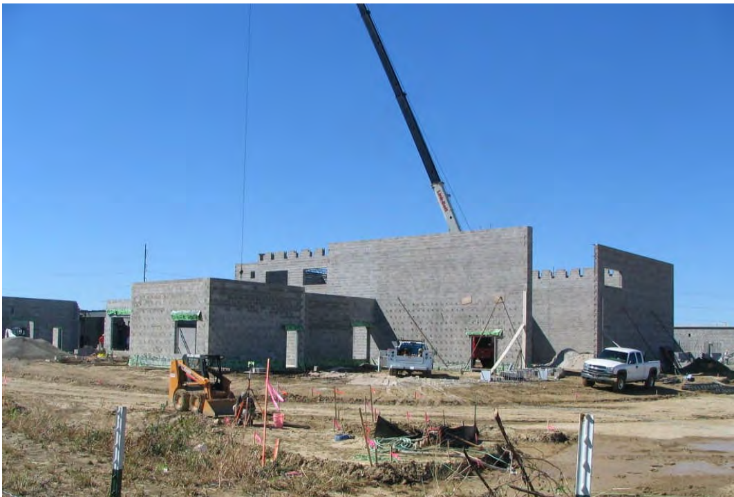
Upchurch Elementary #25 Steel erection at gymnasium continues (October 3, 2007)
