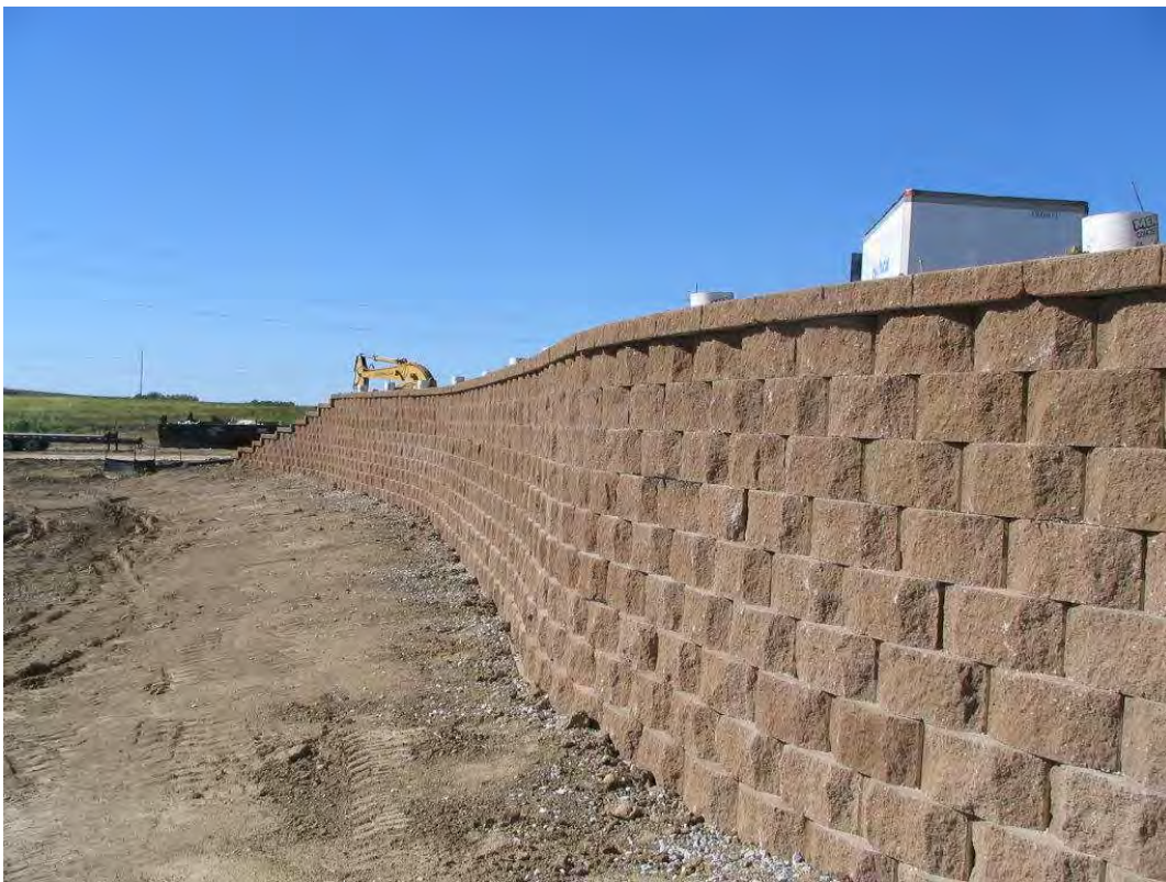
Upchurch Elementary #25 Structural Retaining wall complete (October 3, 2007)
