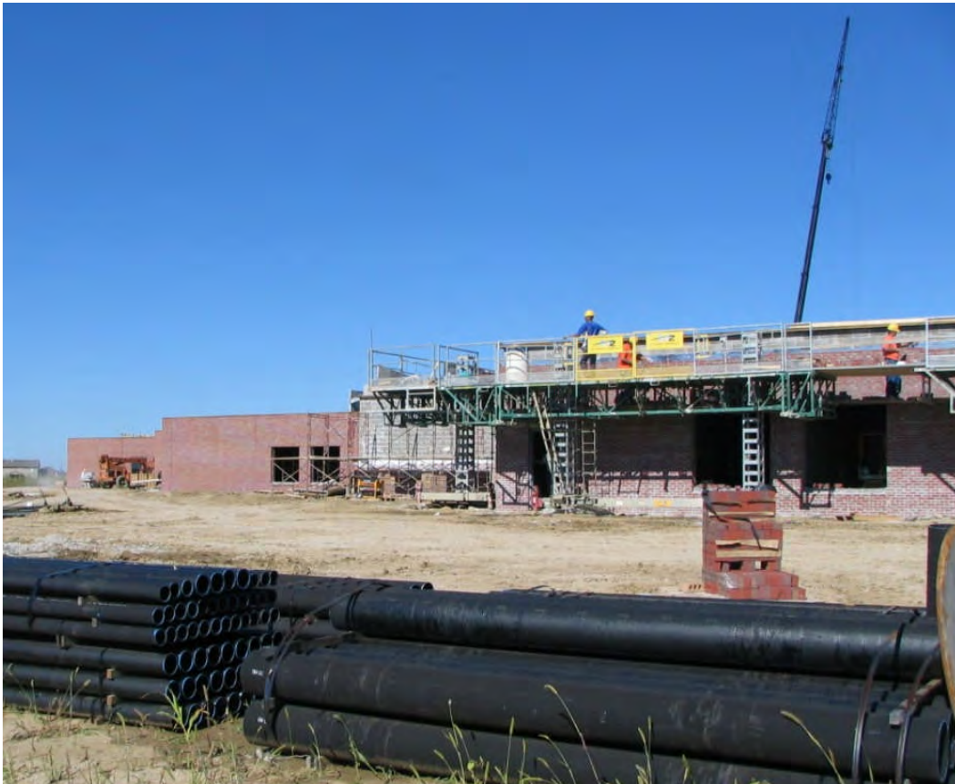
Upchurch Elementary #25 Masonry work in progress (October 3, 2007)
