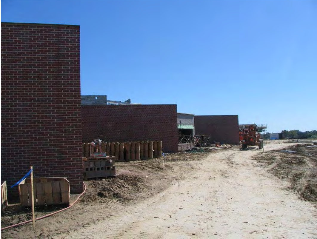
Upchurch Elementary #25 Brick installation west side (October 3, 2007)
