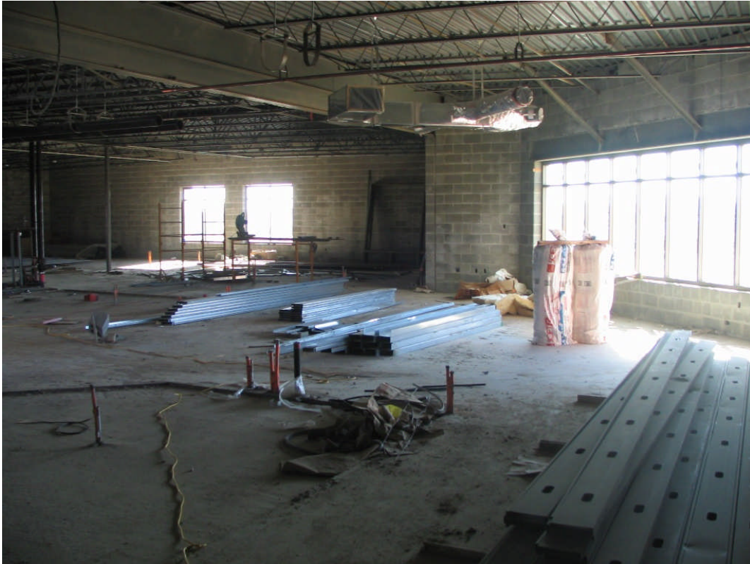
Upchurch Elementary #25 interior construction work underway (Nov 09, 2007)
