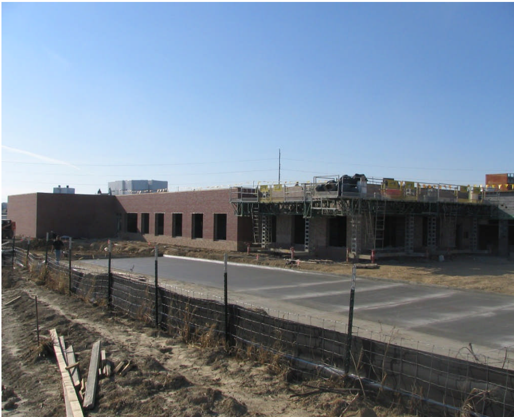
Upchurch Elementary #25 masonry work at front entry (Nov 09, 2007)
