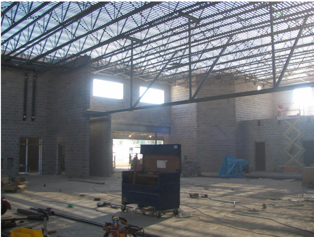
Upchurch Elementary #25 gymnasium/all purpose rooms (Nov 09, 2007)
