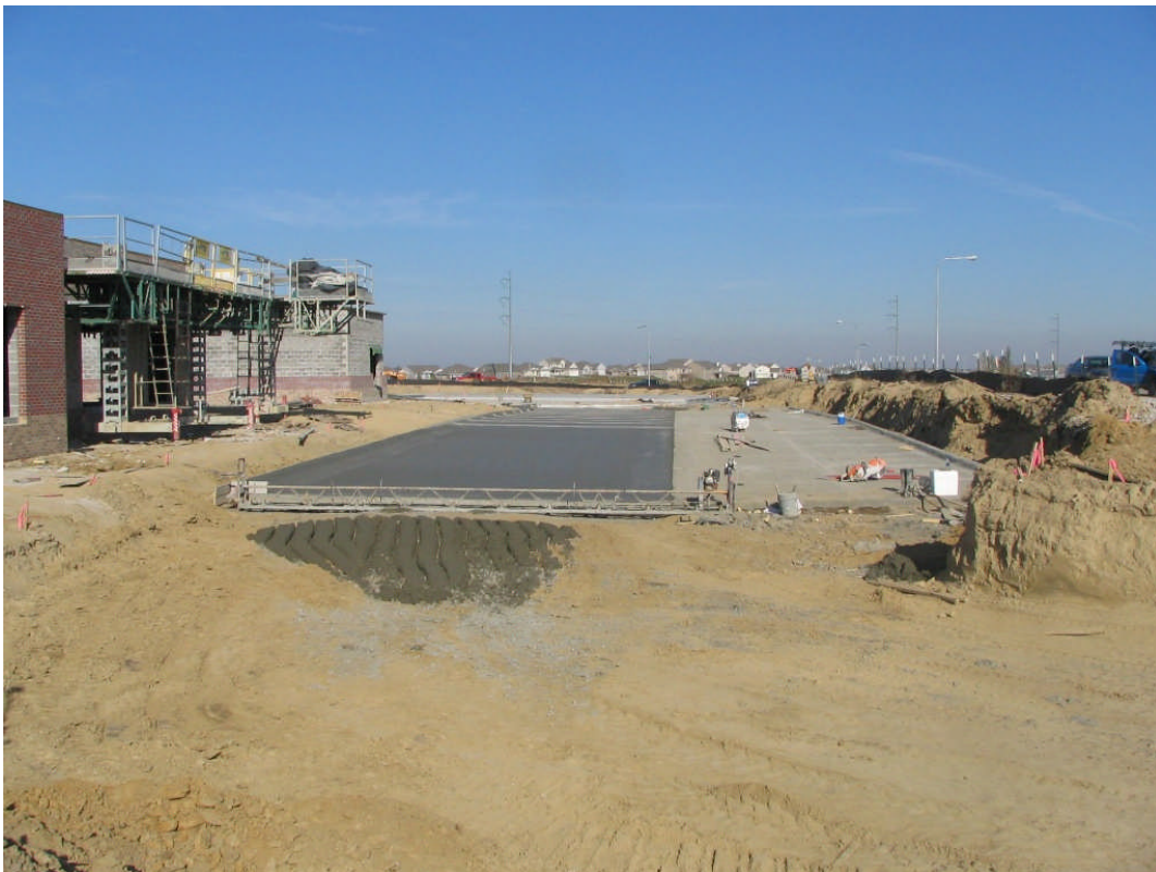
Upchurch Elementary #25 parking paving work in progress (Nov 09, 2007)
