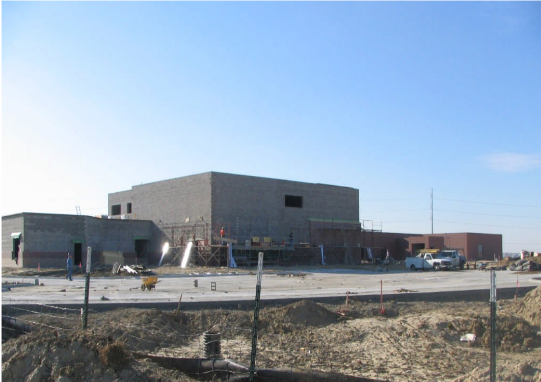
Upchurch Elementary #25 Northeast corner of building (Nov 09, 2007)
