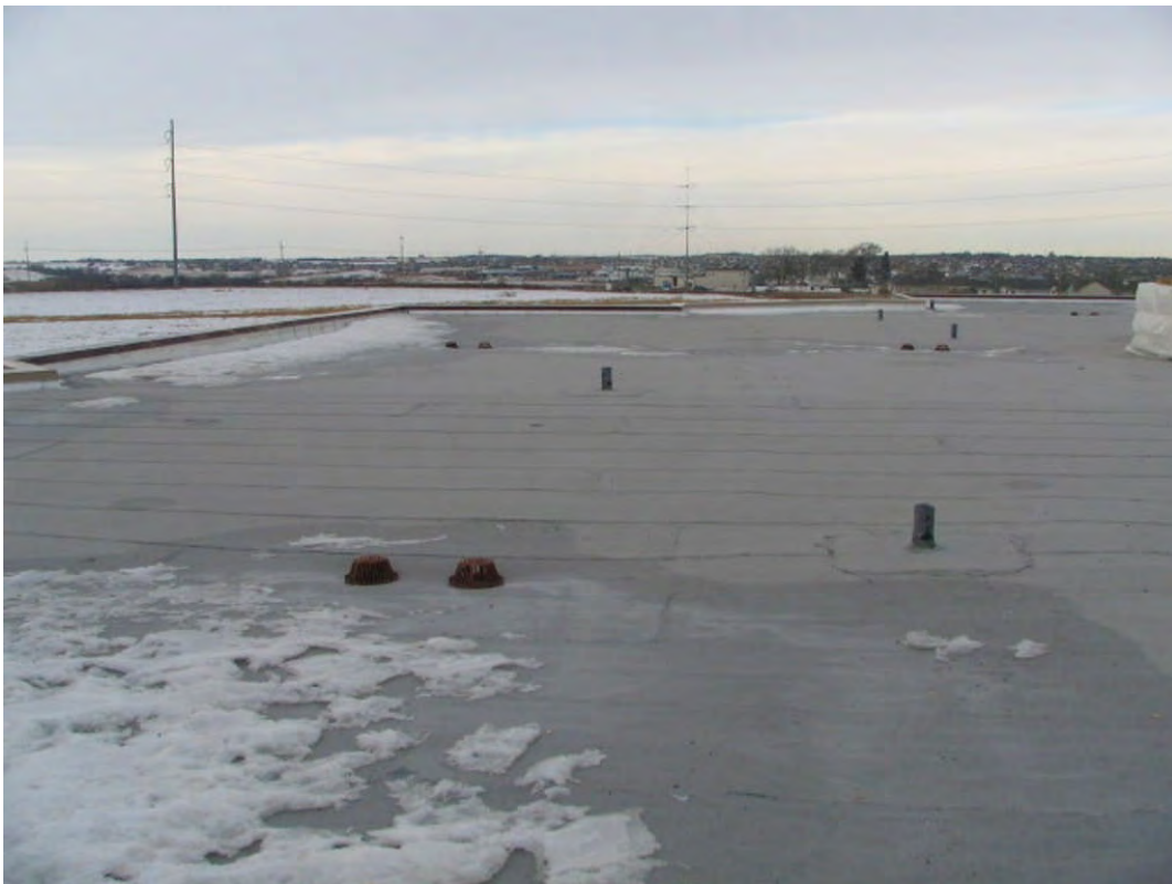
Upchurch Elementary #25 Roofing 'Dried-In' and progressing (Jan 09, 2008)
