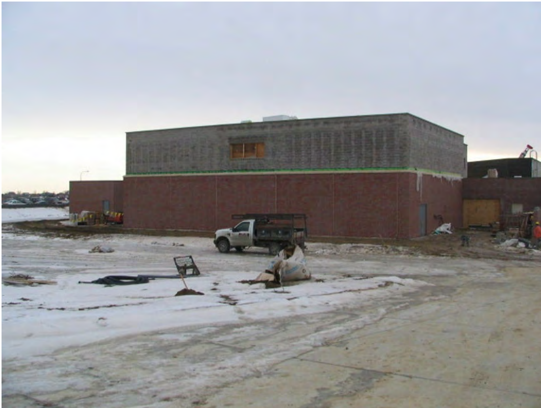
Upchurch Elementary #25 North side of building (Jan 09, 2008)
