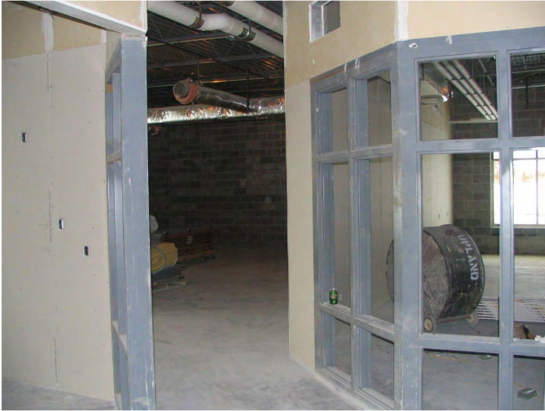
Upchurch Elementary #25 Drywall installation & finishes continue (Jan 09, 2008)
