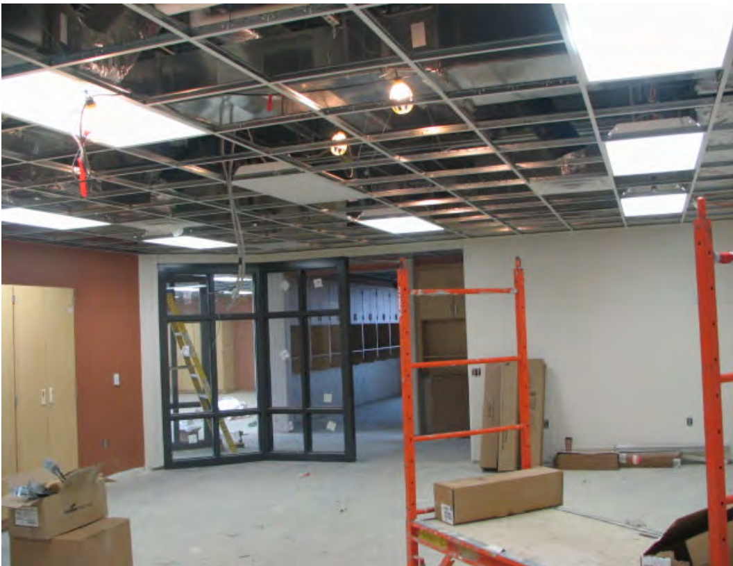
Upchurch Elementary #25 Typical Classroom progress (April 02, 2008)
