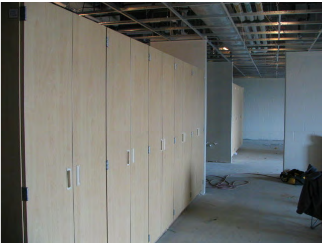
Upchurch Elementary #25 Cabinetry installation @ Kindergarten (April 02, 2008)
