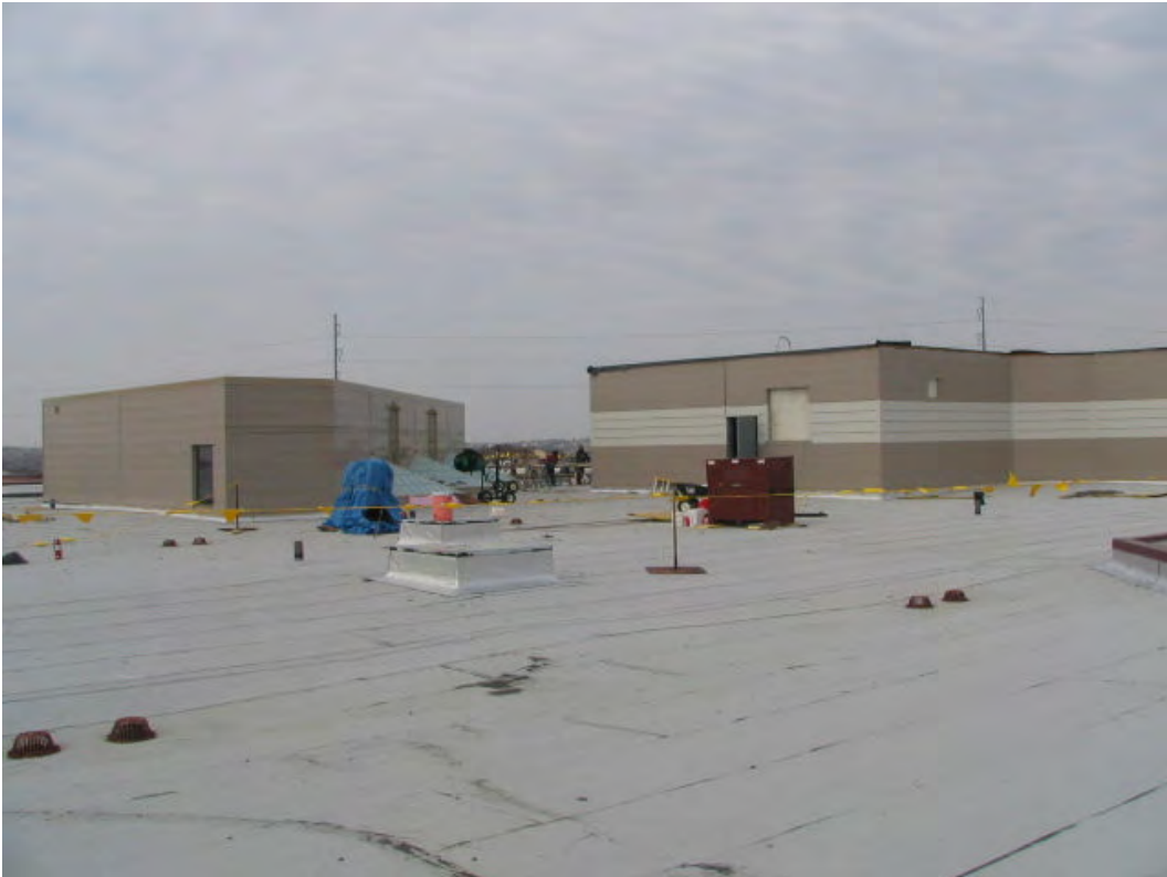
Upchurch Elementary #25 Exterior Metal Panel & Roof (April 02, 2008)
