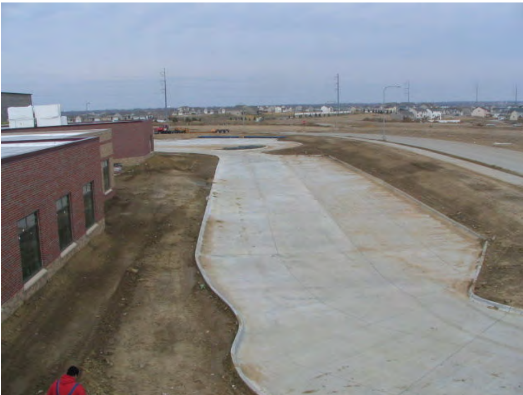
Upchurch Elementary #25 Site grading in progress (April 02, 2008)
