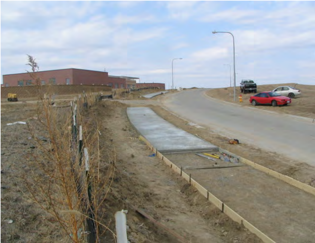
Upchurch Elementary #25 Sidewalk installation started (April 02, 2008)
