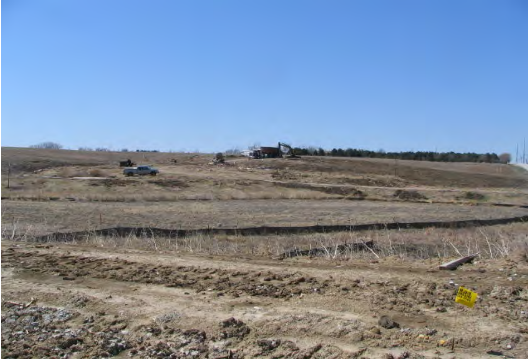
Horizon High School Demolition nearing completion (April 14, 2008)
