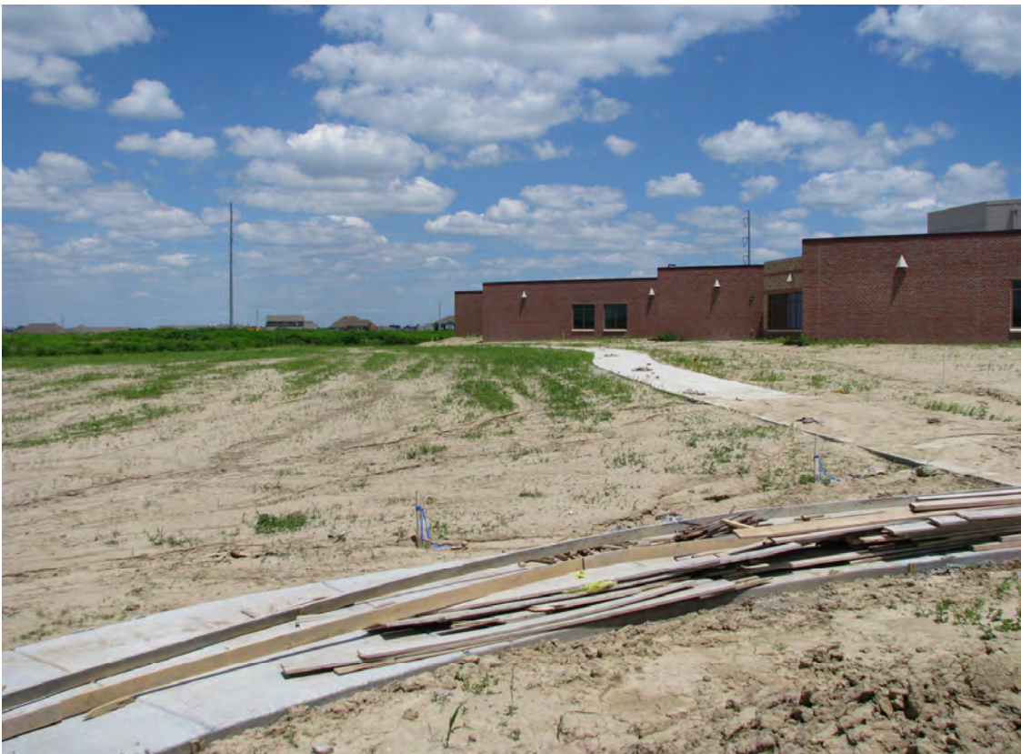
Upchurch Elementary #25 Sidewalk installation (June 30, 2008)
