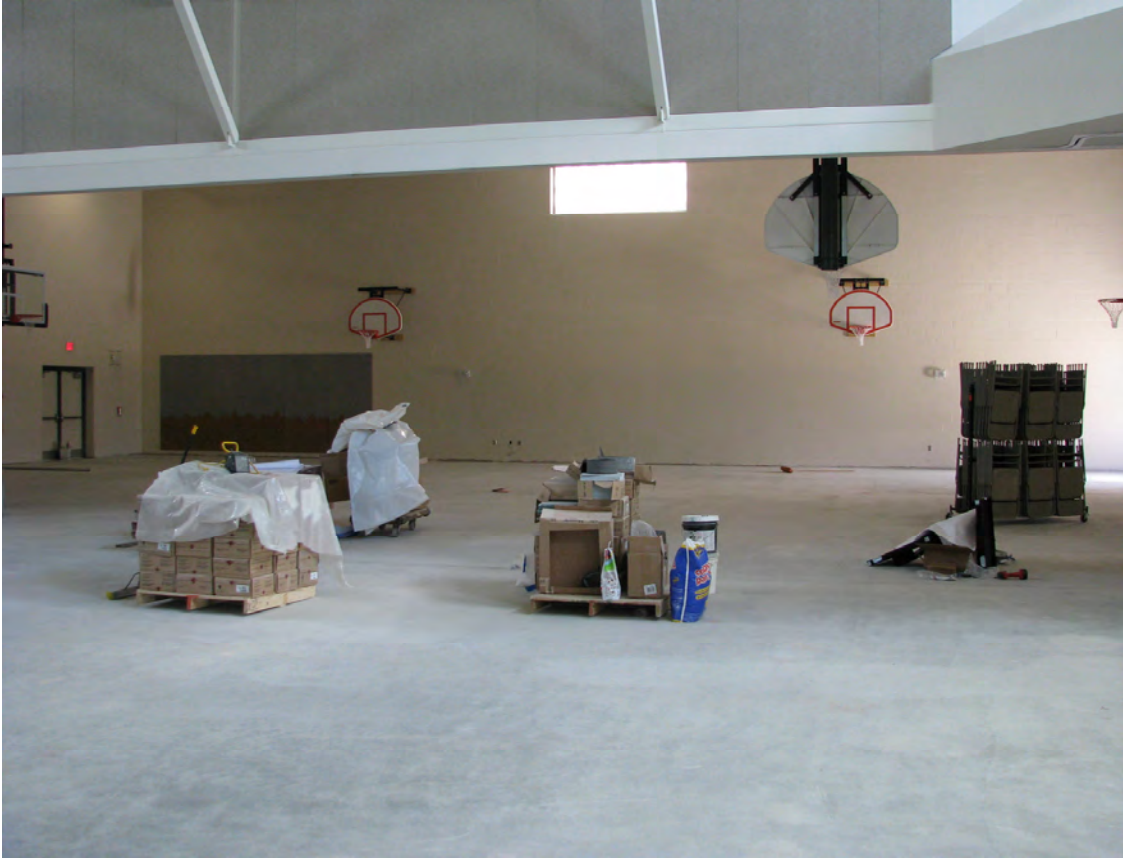
Upchurch Elementary #25 Flooring at Multipurpose & Gymnasium (June 30, 2008)
