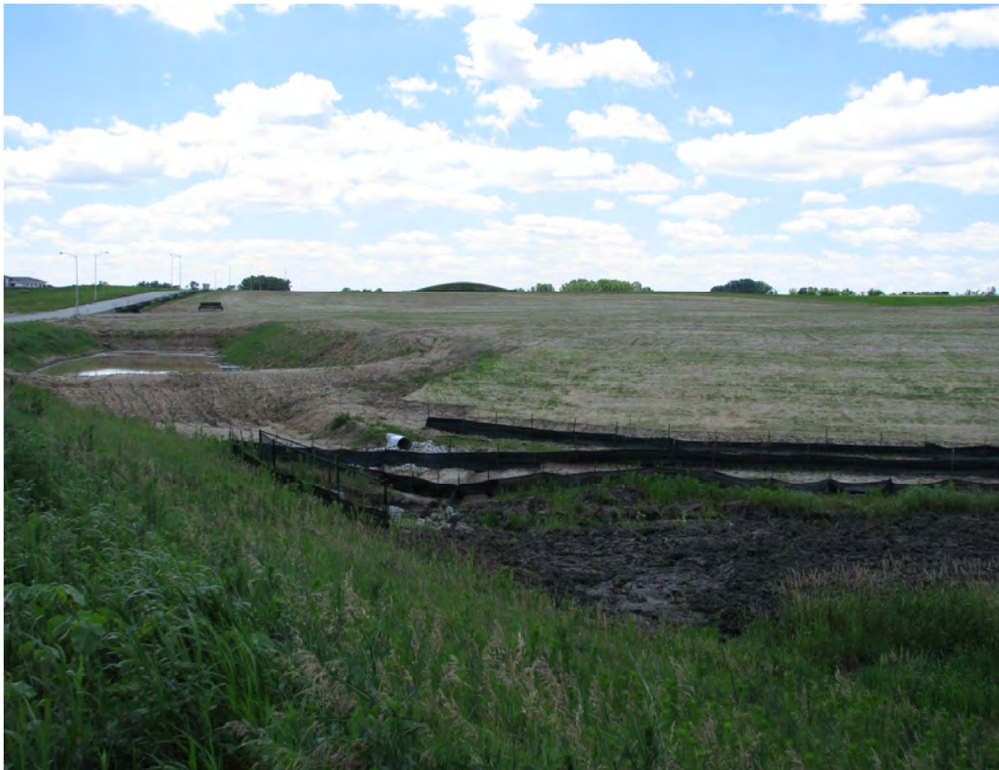
Horizon High School Site Preparation Complete (June 30, 2008)
