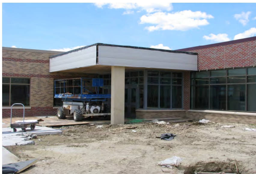
Upchurch Elementary #25 Entrance Canopy (June 30, 2008)
