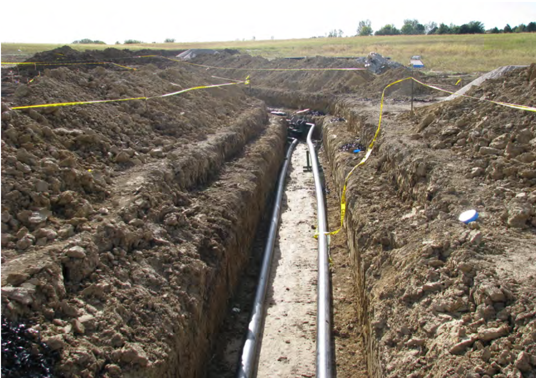
Horizon High School – Geothermal well field connection (Sept 29, 2008)
