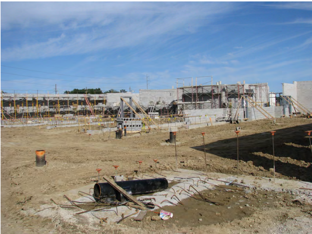
Horizon High School – Interior wall construction (Sept 29, 2008)
