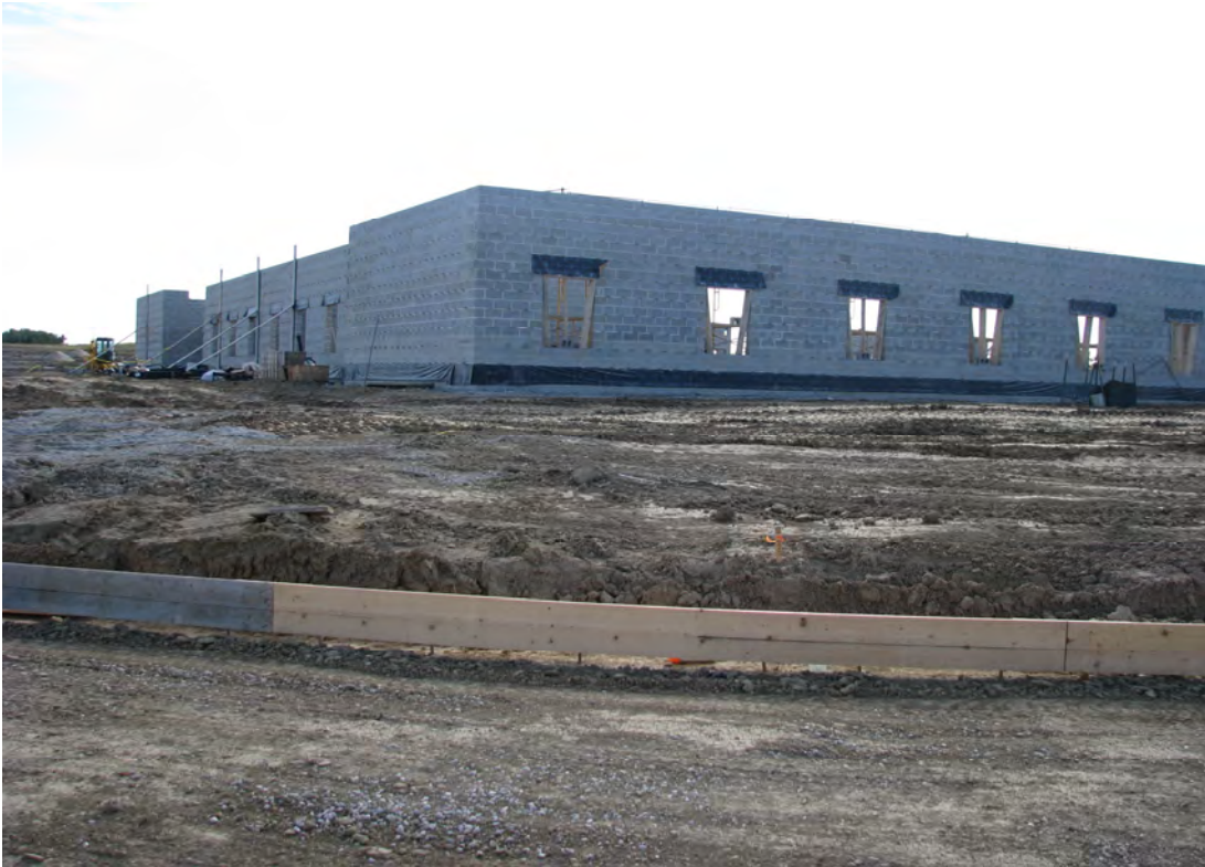
Horizon High School – Masonry wall installation (Sept 29, 2008)
