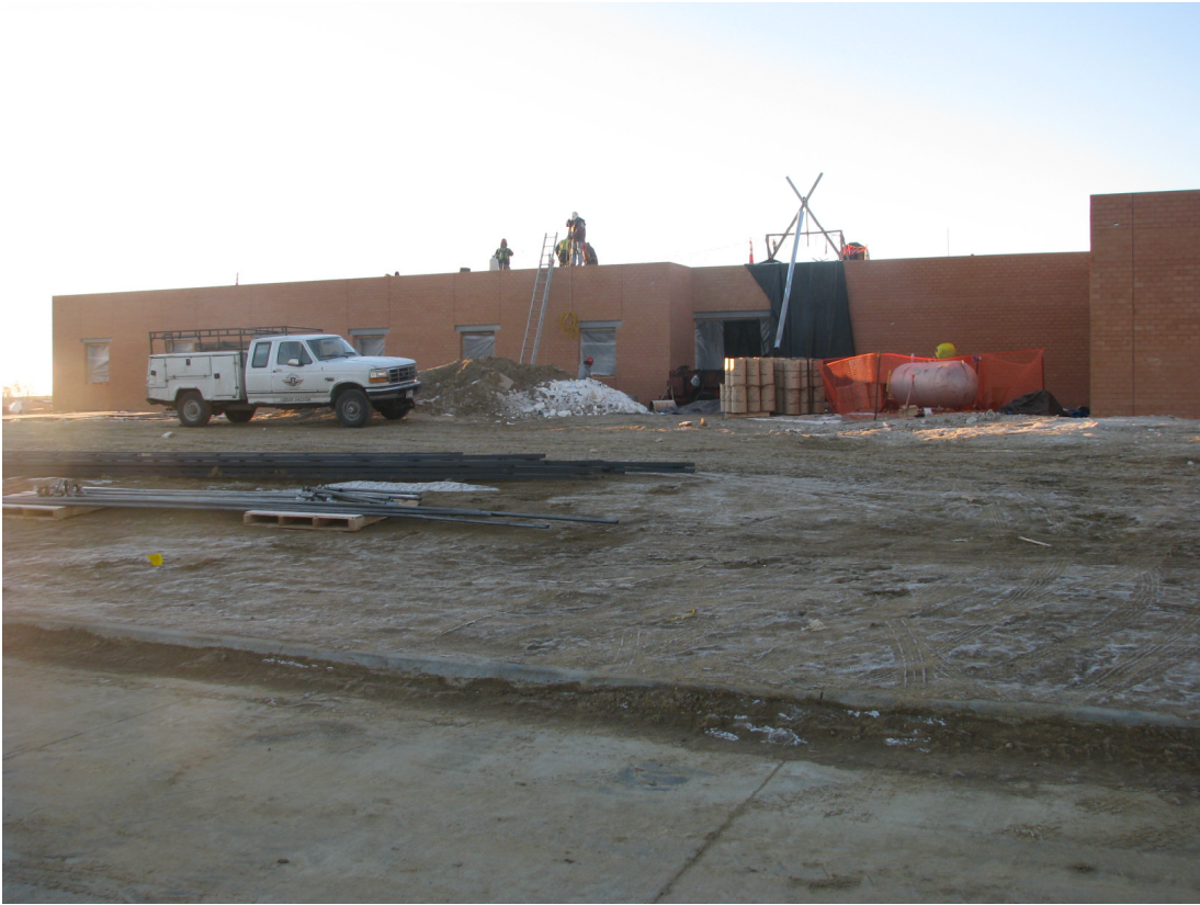
Horizon High School – Exterior brick and roofing installation (Jan 21, 2009)
