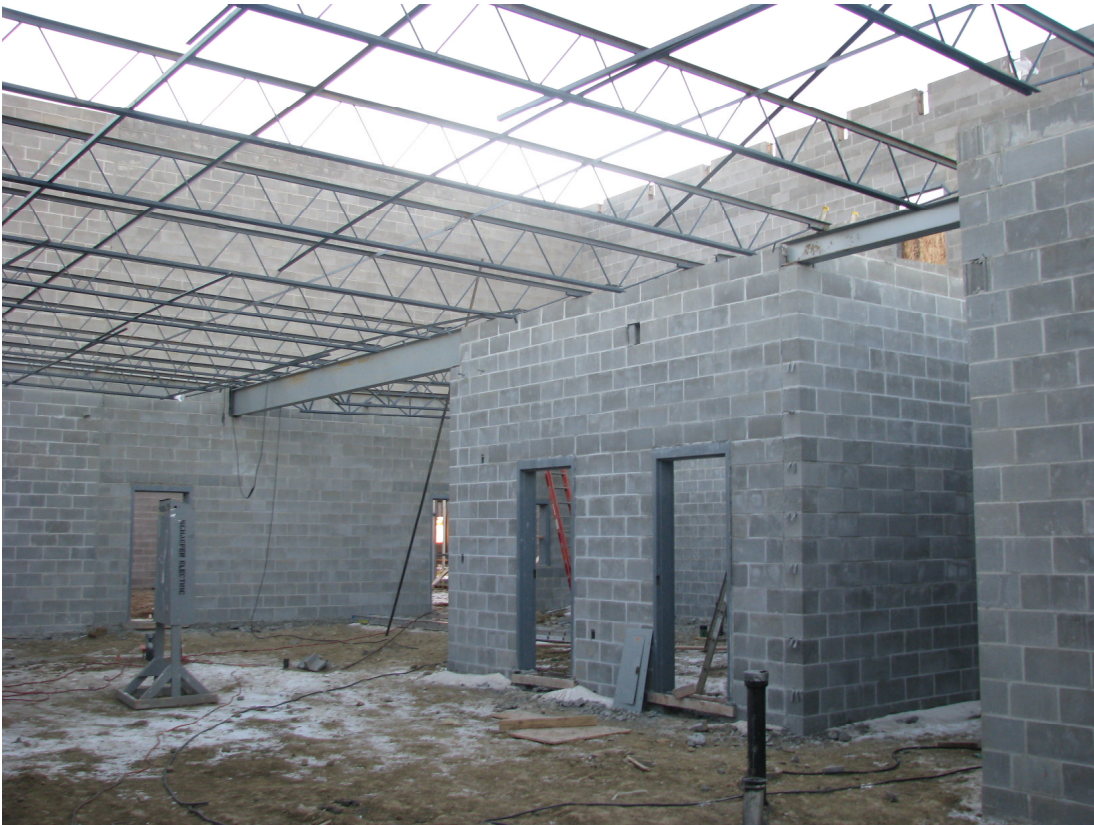
Horizon High School – Steel joists installation (Jan 21, 2009)
