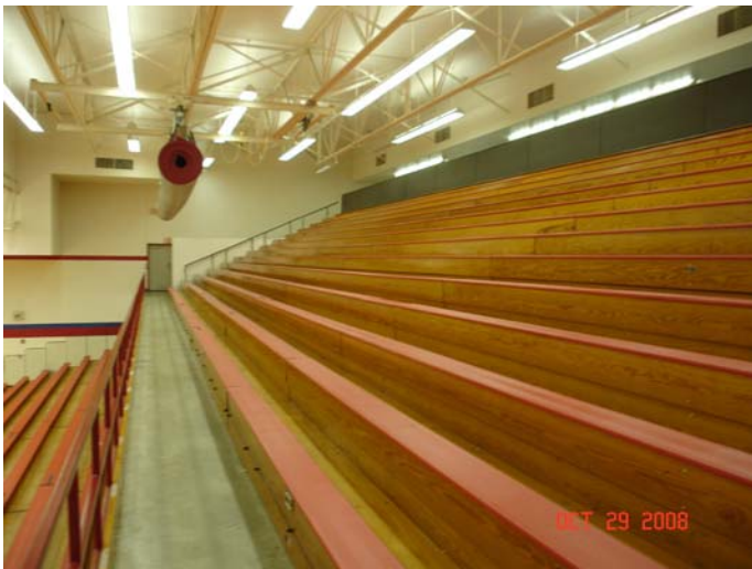
Mezzanine Level – Old Rails
