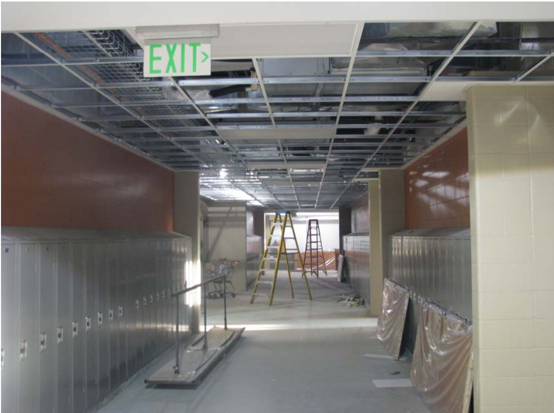
Horizon High School – Typical Corridor (October 1, 2009)
