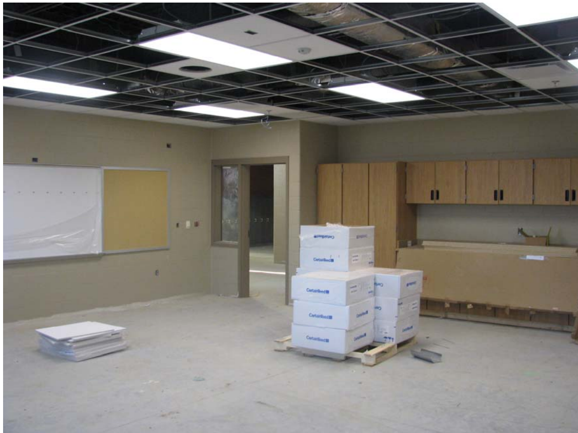
Horizon High School – Typical Classroom (October 1, 2009)
