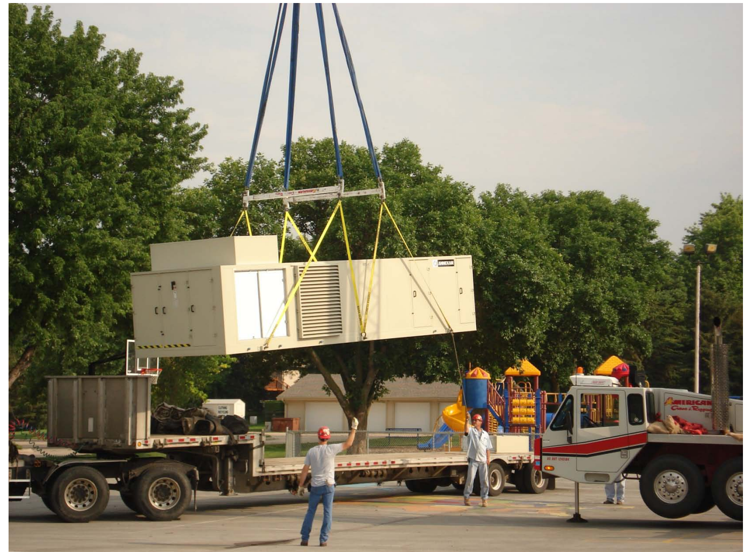
RTU Being Hoisted to Roof at Sandoz in 2007
